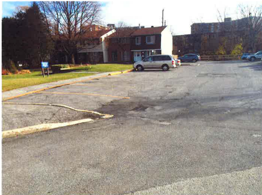
2 Showing the condition of the asphalt pavement in the rear parking lot. Note cracking and heaving
