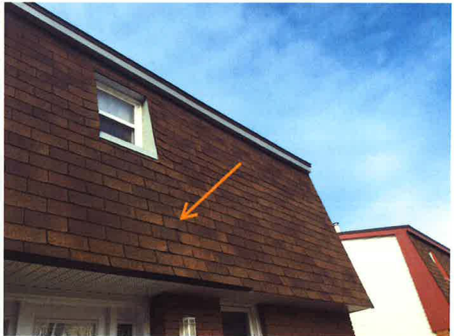
10 Showing typical condition of the asphalt shingle mansard roofs. Note minor uplift.
