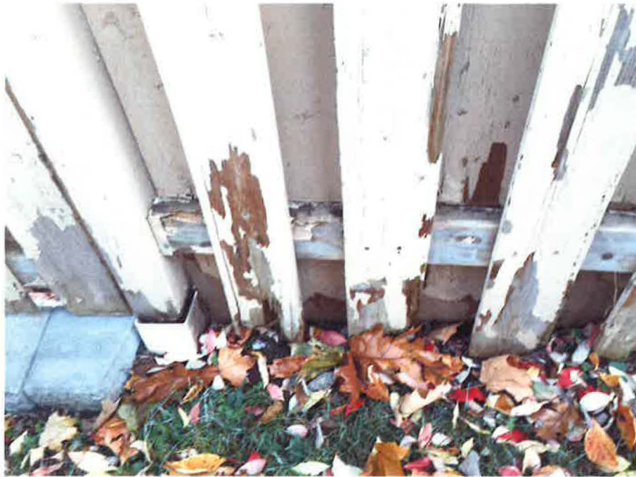
5 Showing a section of deteriorated wood fencing
