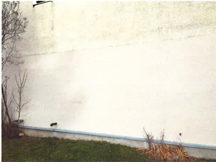
7 Showing existing cracked stucco to be replaced with vinyl siding
