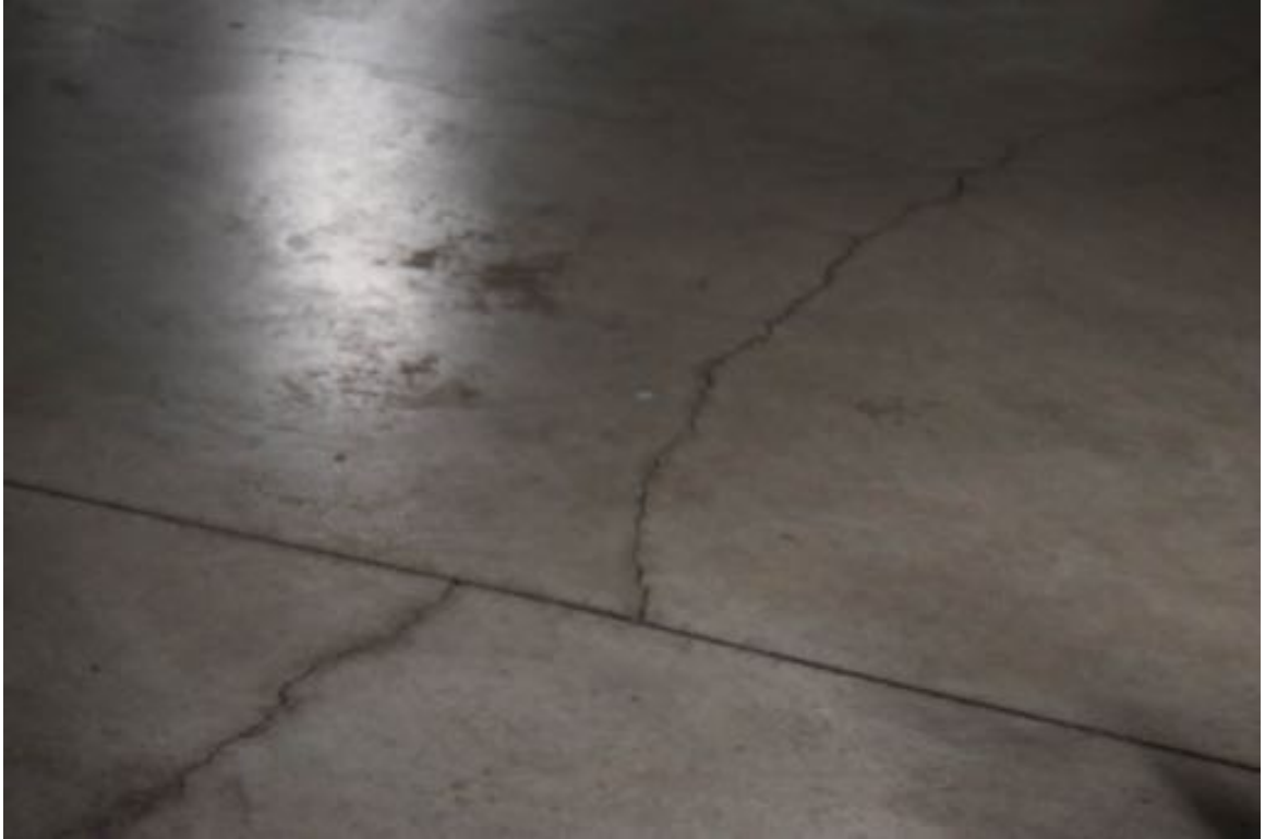
Photo 25: There are various size cracks in the cement slab at multiple locations.
