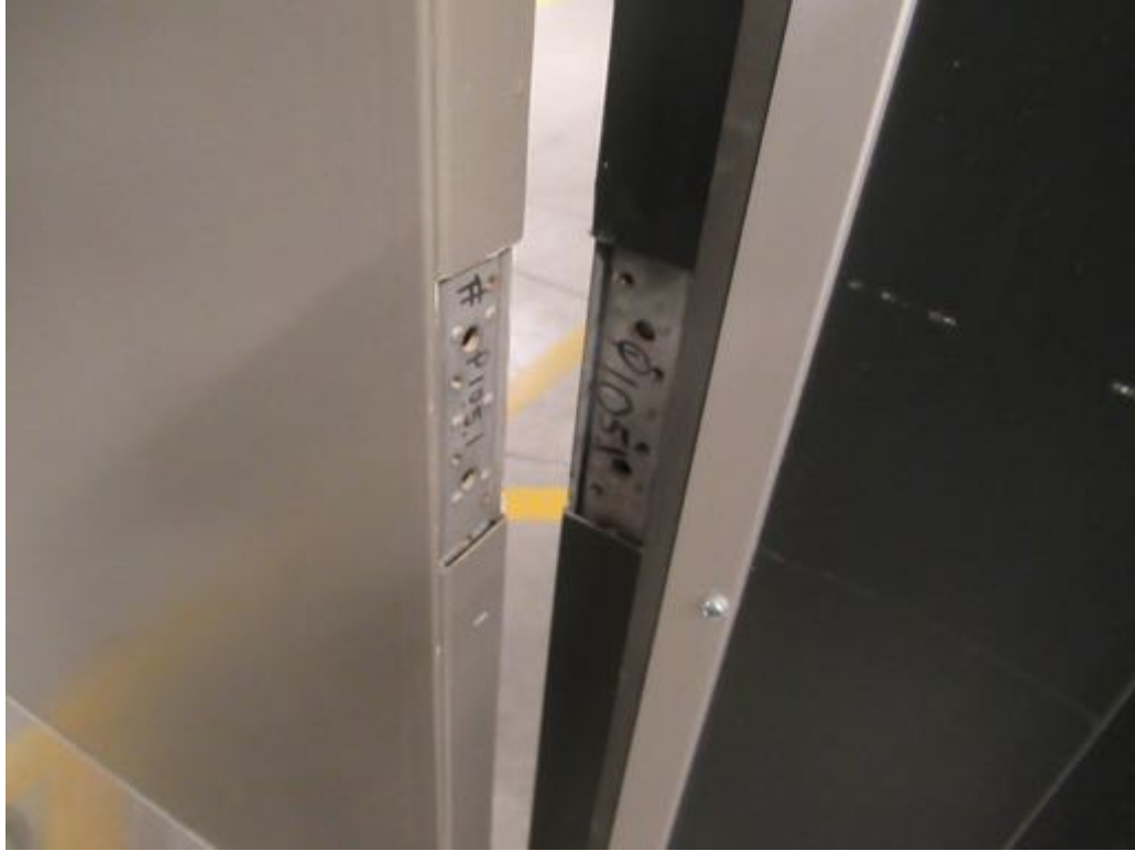
Photo 87: Garbage room door is missing some hinges.
