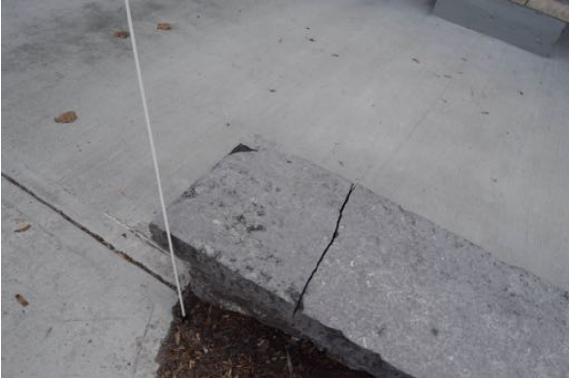
Photo 1: For the small retaining wall leading up to the ramp entrance, the top masonry cap has a large crack, and a chipped corner.
