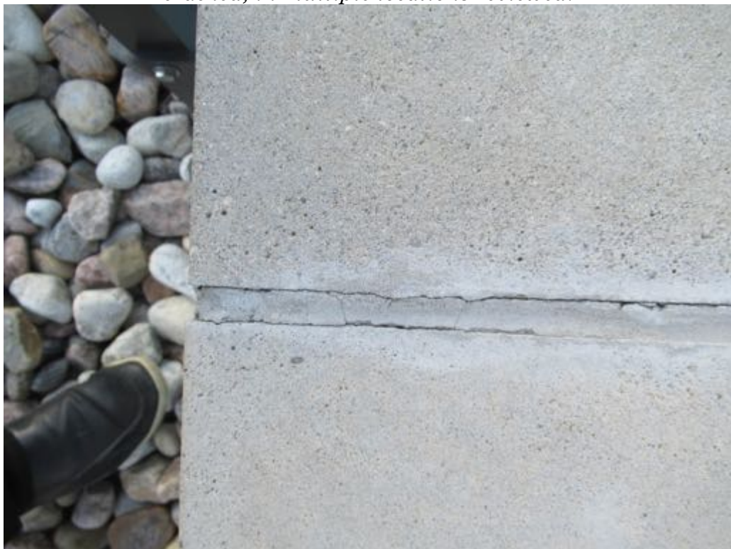
Photo 68: The mortar between the fourth floor terraces precast concrete caps is cracked, in multiple locations reviewed.
