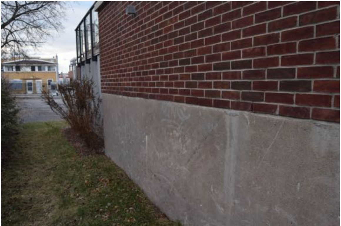
Photo 20: The southeast corner above grade foundation wall appears to be from the old existing building, and not new construction.
