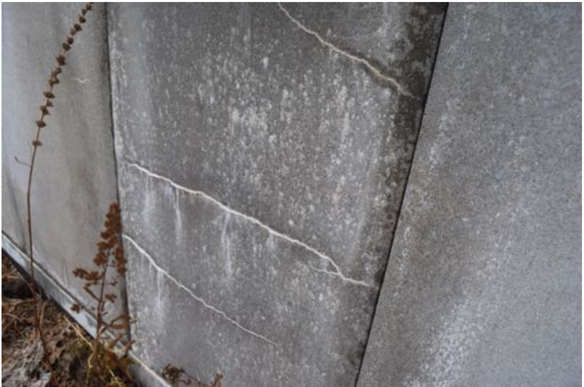
Photo 50: Multiple cracks are visible in the panels, particularly under the scuppers.
