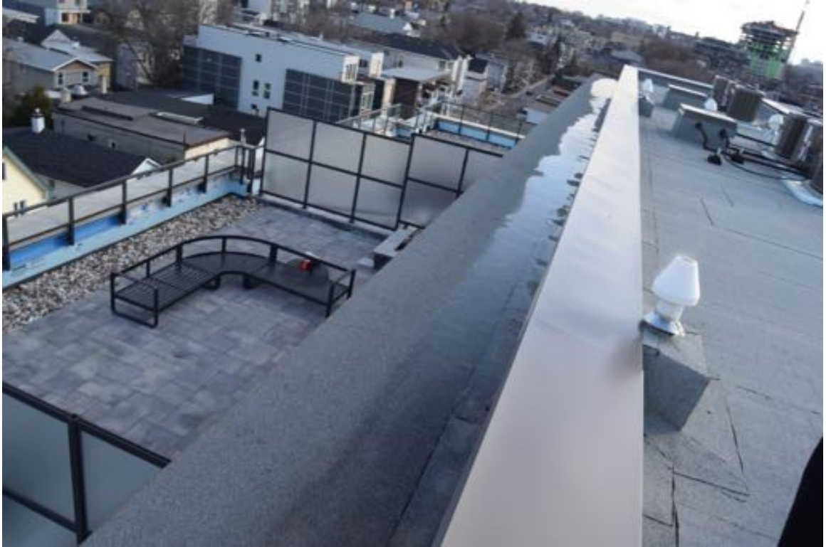
Photo 61: For the majority of this eyebrow roof, there was standing frozen water observed.
