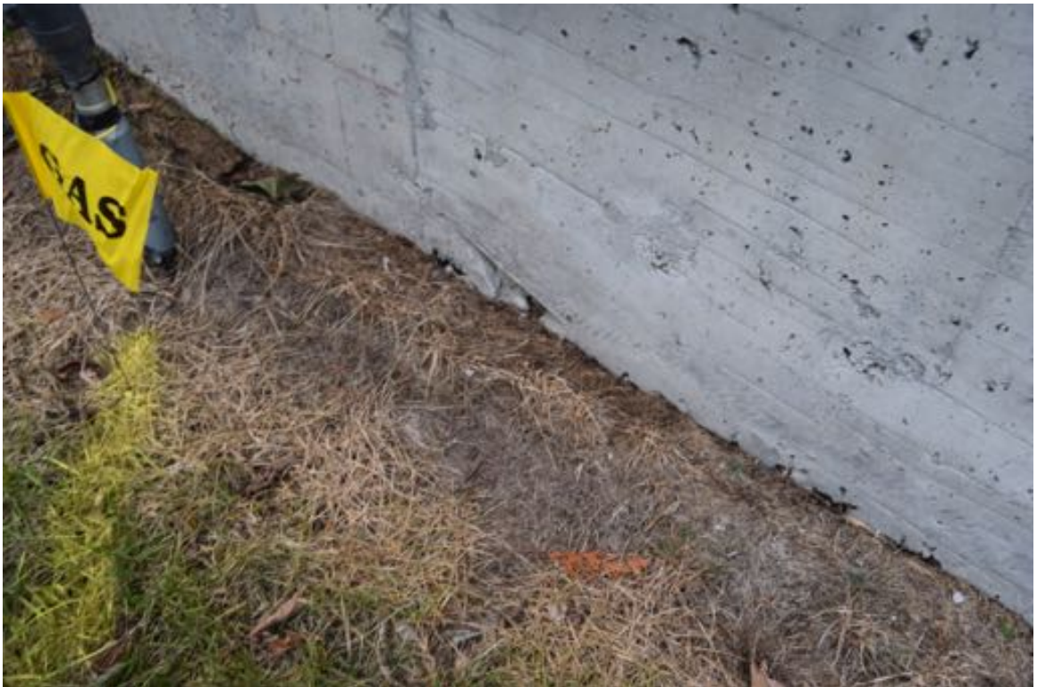
Photo 14: Southeast side, foundation honeycombing near grade.
