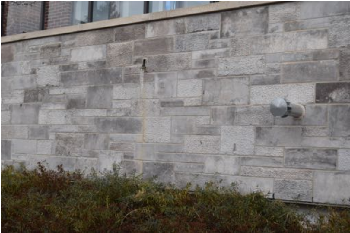
Photo 52: East elevation, the masonry veneer cladding of north terrace has staining/discolorations under the scupper.
