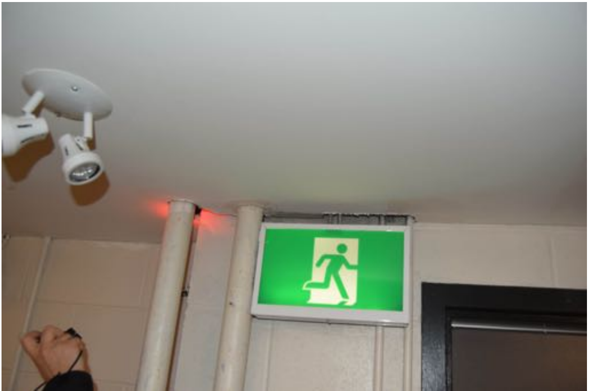
Photo 80: In a number of areas, there are open gaps in the ceilings, particularly around pipe and conduit penetrations.
