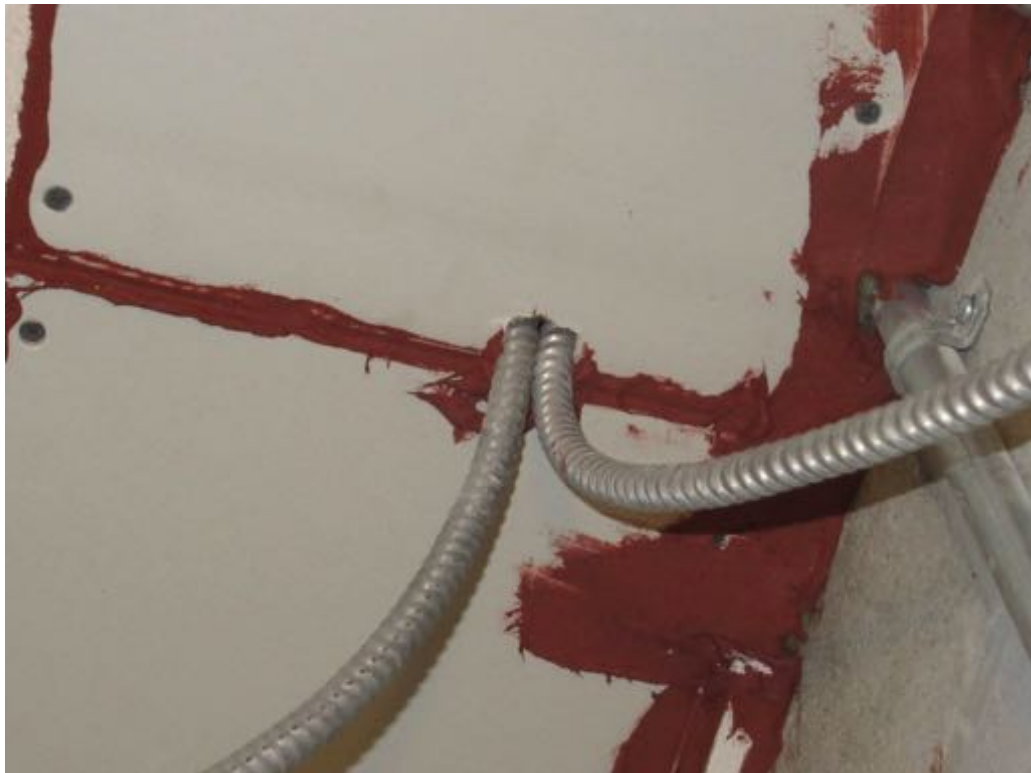
Photo 74: In the elevator control room, firestopping is missing around a ceiling penetration .
