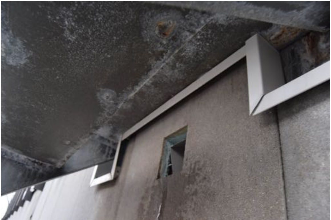
Photo 48: At the west elevation, scupper appears draining behind a panel, causing deterioration between panels near an exhaust vent.
