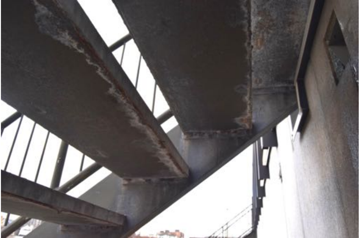
Photo 3: South staircase is rusting at the bottom.
