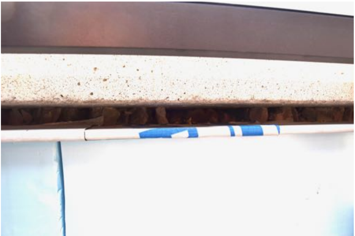
Photo 66: The mortar under the precast concrete caps on fourth floor terraces appears to be missing/deficient in multiple areas.
