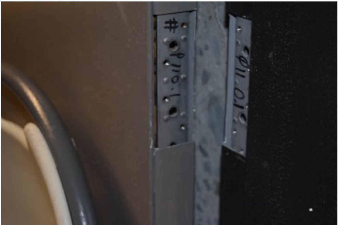
Photo 88: Unit storage room doors have hinges missing.
