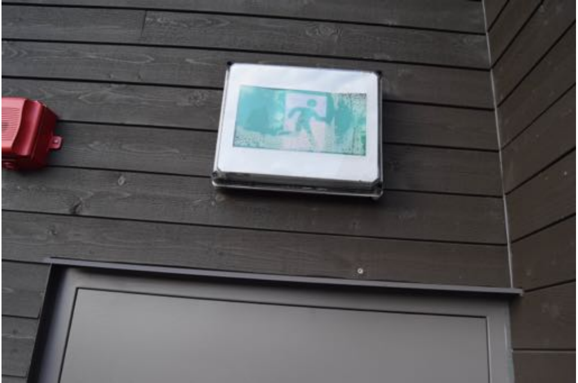
Photo 75: Condensation in protective enclosure of the exit sign at fourth floor common terrace.
