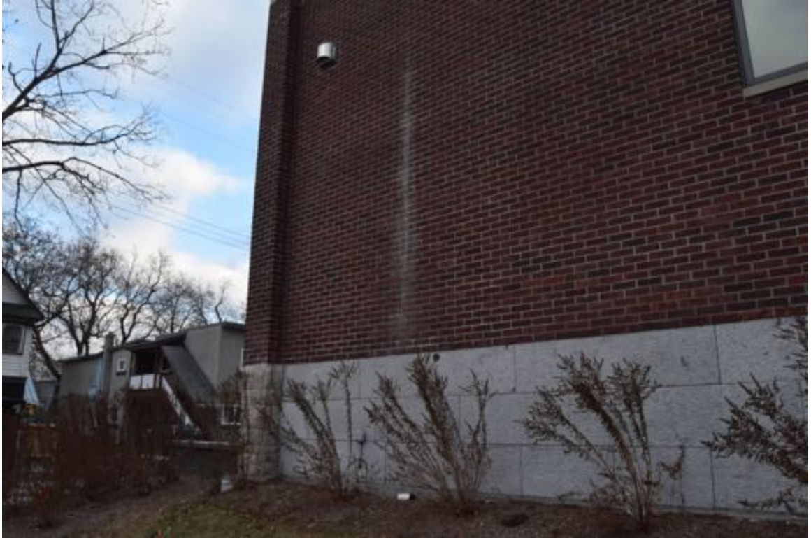
Photo 35: North elevation, significant staining visible from the balcony scuppers on the brick veneer.
