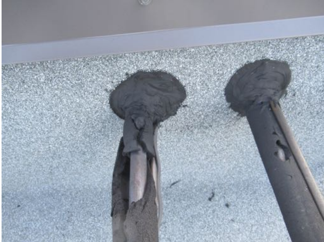
Photo 71: Piping insulation is deteriorating at certain locations.
