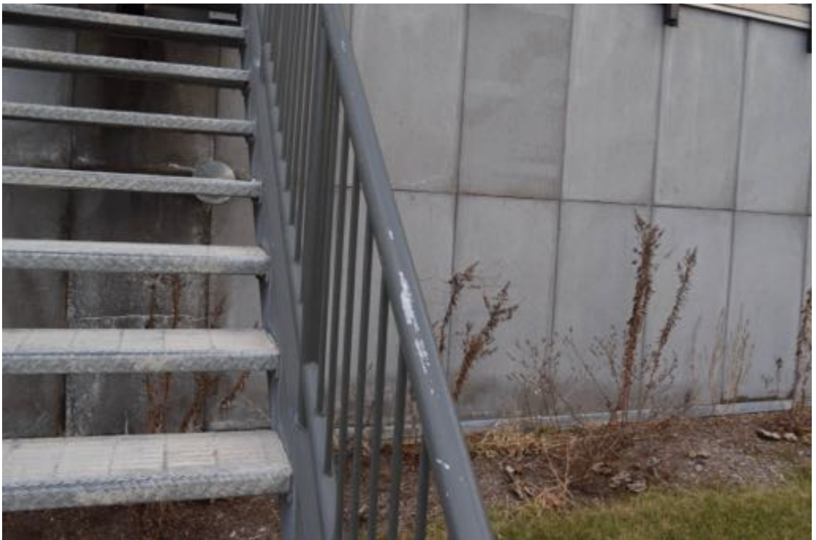
Photo 4: Paint is peeling on the south staircase.
