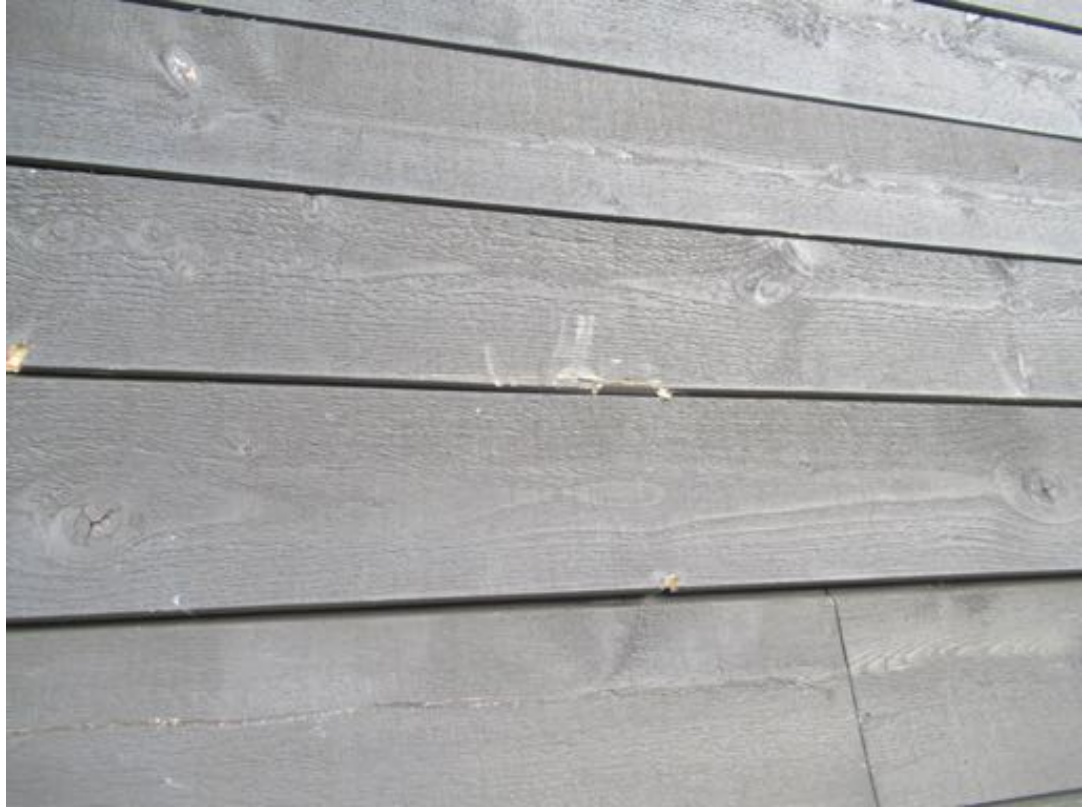
Photo 41: Various dings/scratch marks observed on the wood cladding, at northwest common fourth floor terrace.
