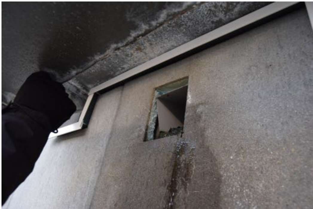
Photo 46: At the west elevation, multiple scuppers for terrace drains do not extend far enough beyond the cement insulation panels, causing heavy staining, ice build-up, and deterioration of the panels.
