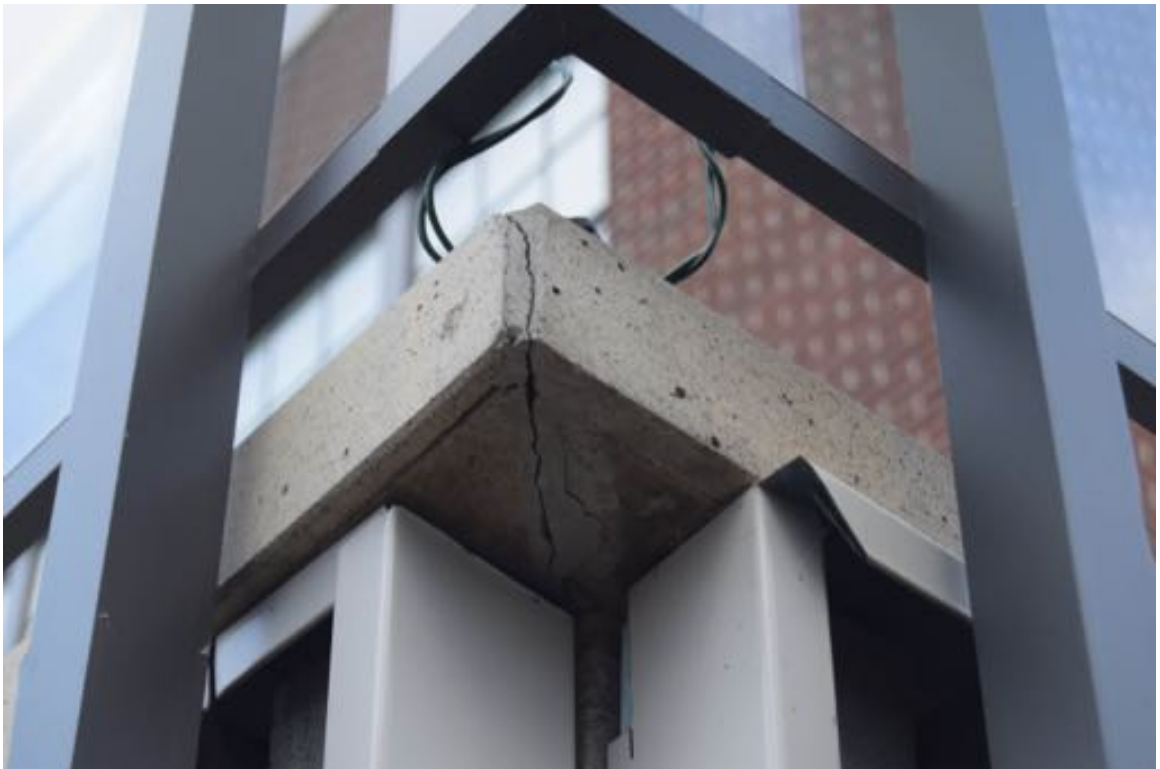
Photo 62: There is a cracked parapet precast cap, south corner of the southwest terrace.
