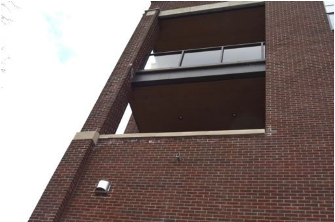
Photo 34: North elevation, discoloration/staining visible on brick veneer under precast elements.
