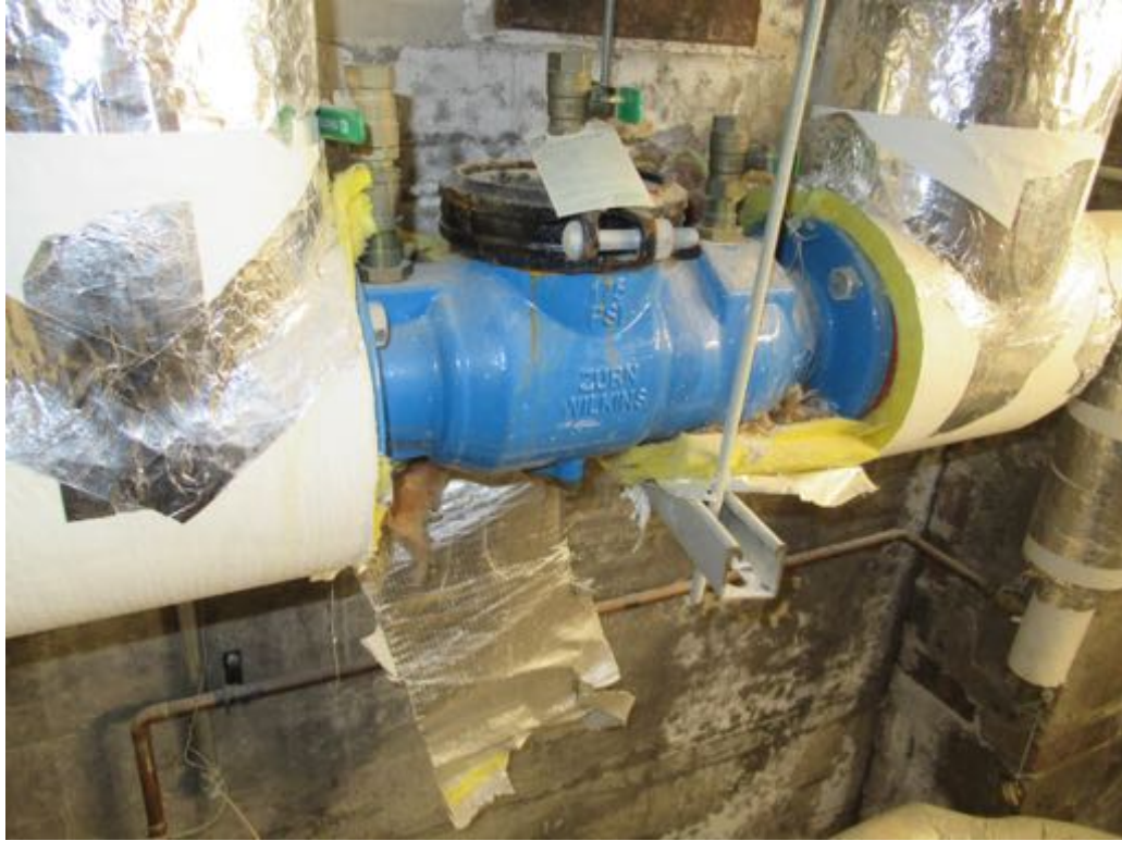
Photo 69: Insulation appears to have been removed from piping in the water entry room, to be reviewed/repared.
