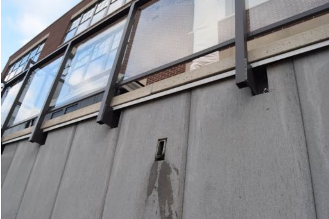
Photo 45: At the west elevation, multiple scuppers for terrace drains do not extend far enough beyond the cement insulation panels, causing heavy staining, ice build-up, and deterioration of the panels.
