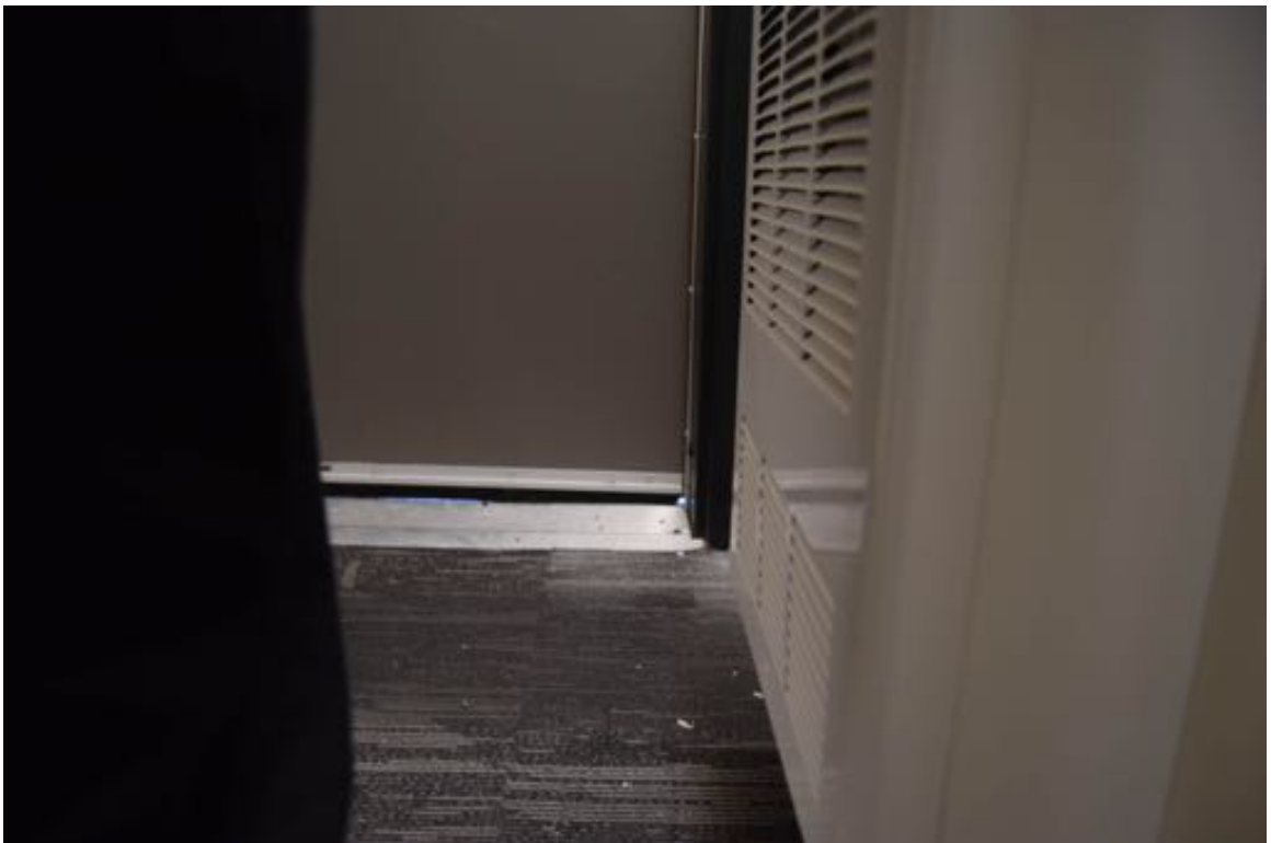
Photo 54: Stairwell C, there is a gap at the bottom of the door to the common fourth floor terrace.
