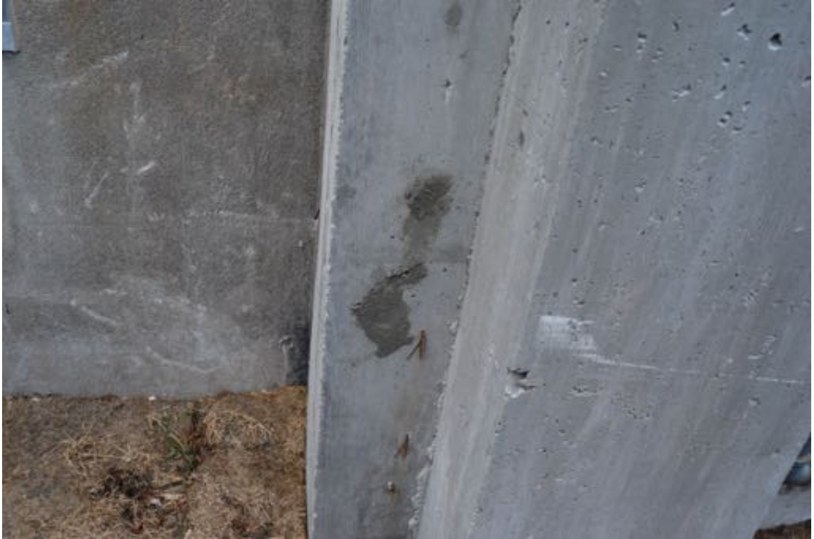
Photo 17: Southeast elevation, rusting nails protruding from the foundation.
