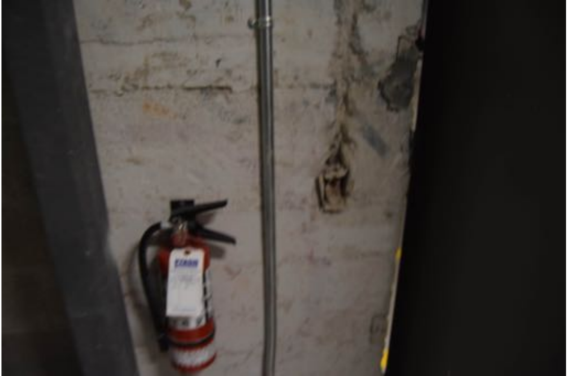
Photo 85: The wall finishes behind the door in the electrical room are poor.
