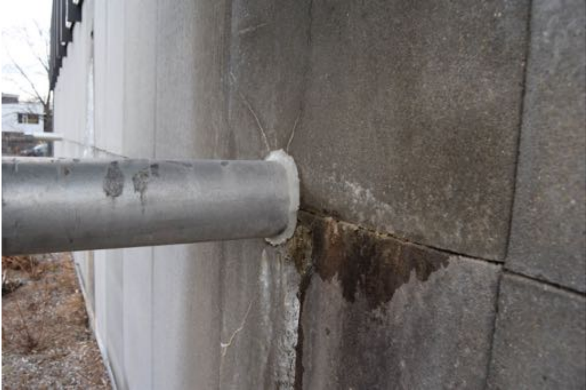
Photo 47: At the west elevation, scupper appears draining behind a panel, causing deterioration between panels near an exhaust vent.
