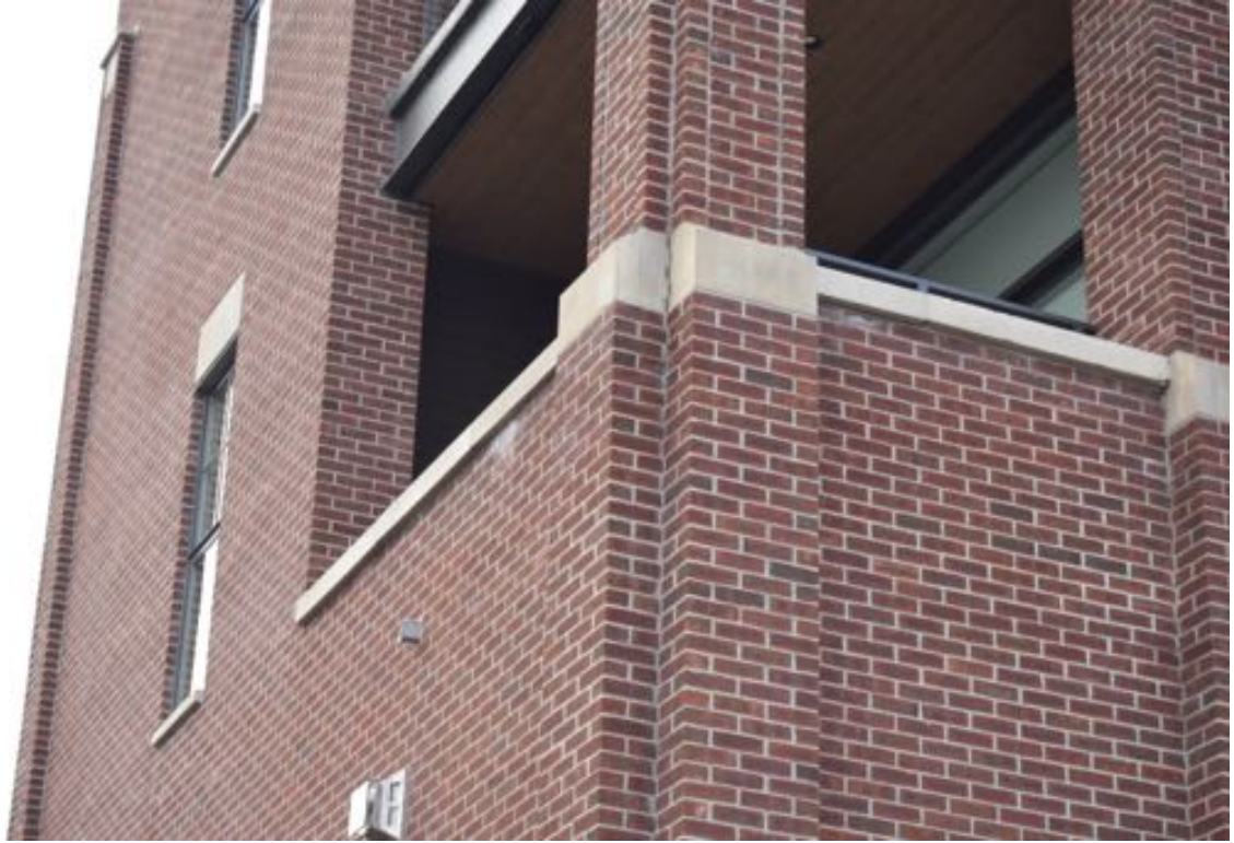
Photo 29: Southeast corner of the building, discoloration/staining visible on brick veneer under balcony precast caps.
