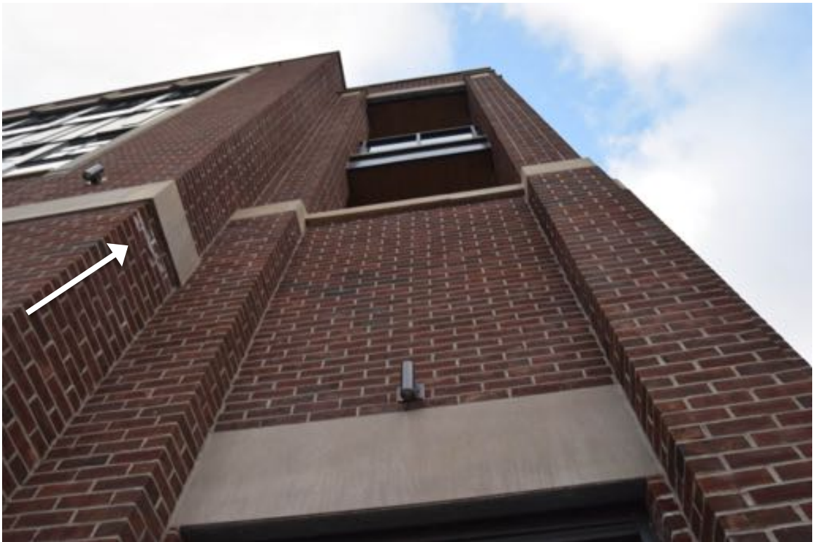
Photo 36: East elevation, northeast corner of the building, discoloration/staining visible under a precast cladding panel.
