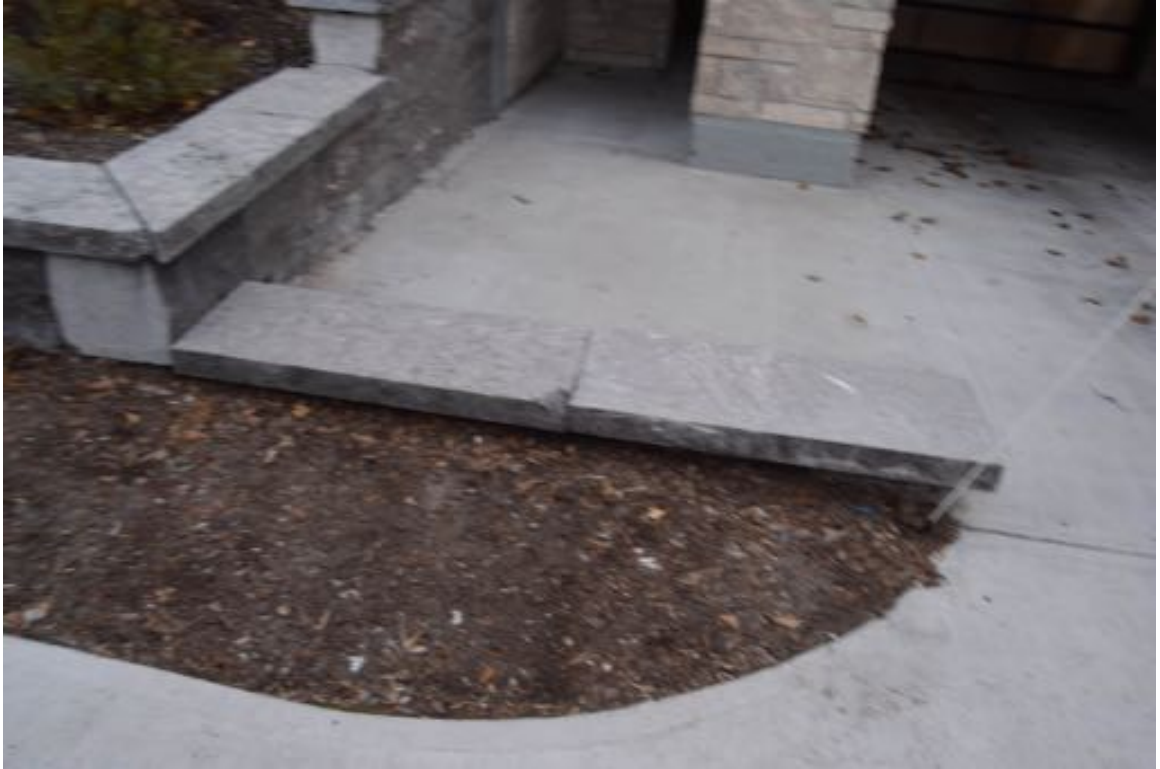
Photo 11: Sod areas adjacent to entrance ramp have sod missing.
