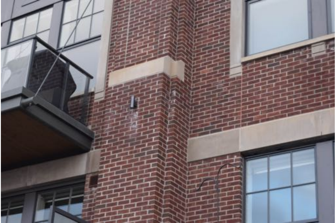
Photo 37: East elevation, there are numerous locations where there is discoloration/staining on the brick veneer, including under precast concrete elements, precast parapet caps, under exterior lighting, etc
