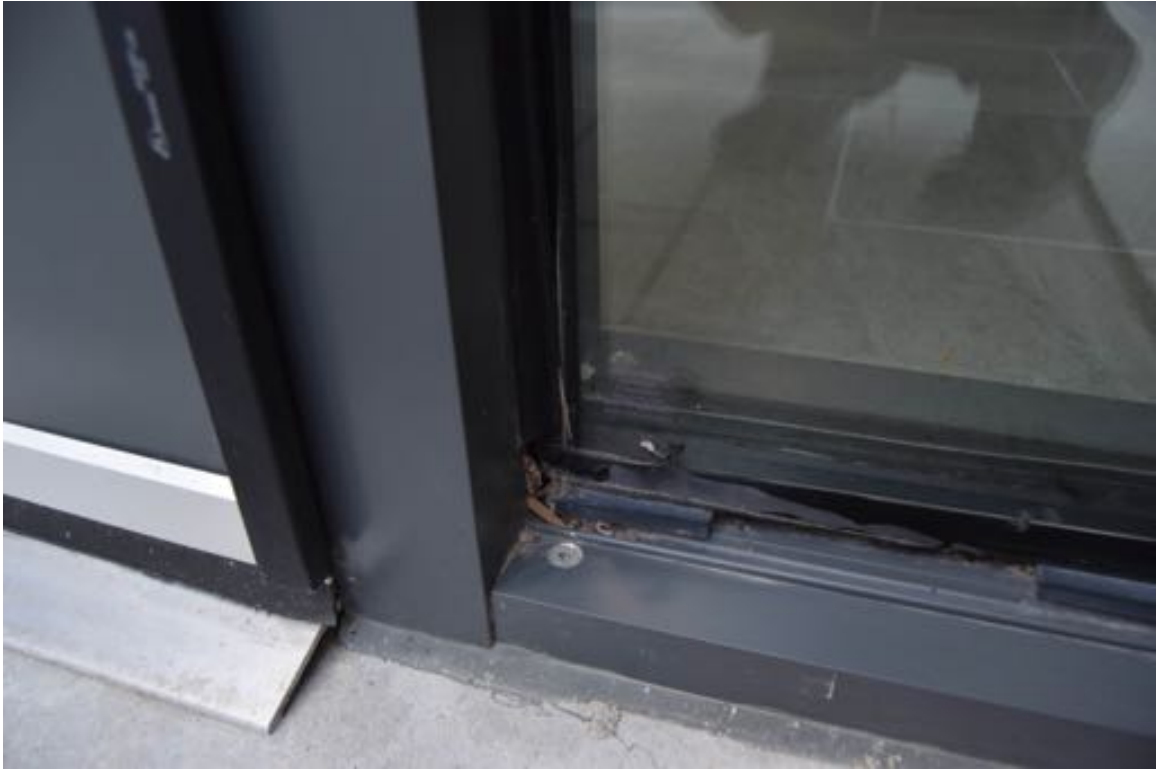
Photo 55: Northeast exterior door to stairwell D, a cap piece is missing.
