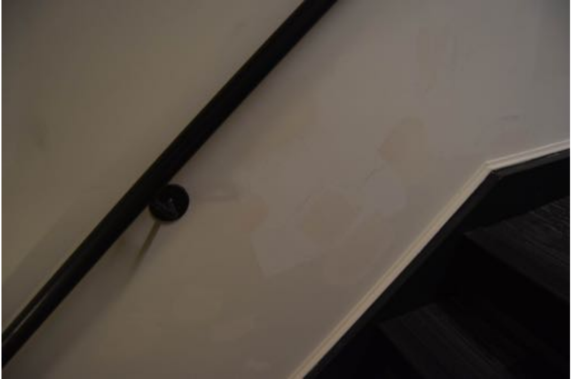
Photo 79: A number of areas where the walls require painting in the stairwells.
