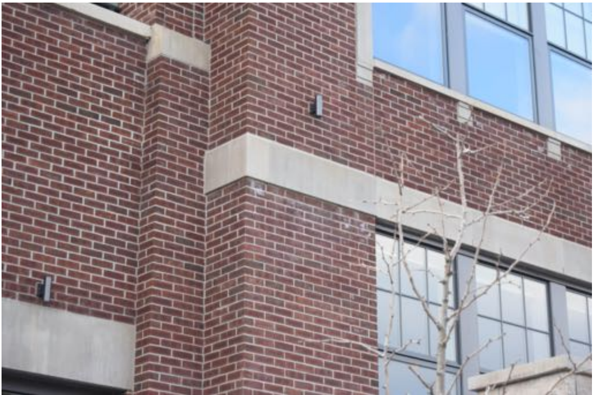
Photo 28: Southeast corner of the building, discoloration/staining visible on brick veneer under precast panels
