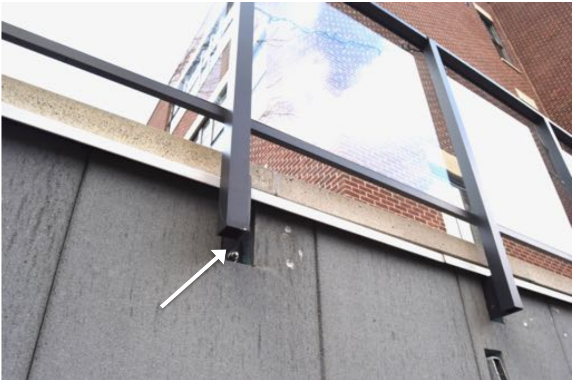
Photo 44: At multiple locations, the insulation is exposed at the connection points of the terrace aluminum guardrails.
