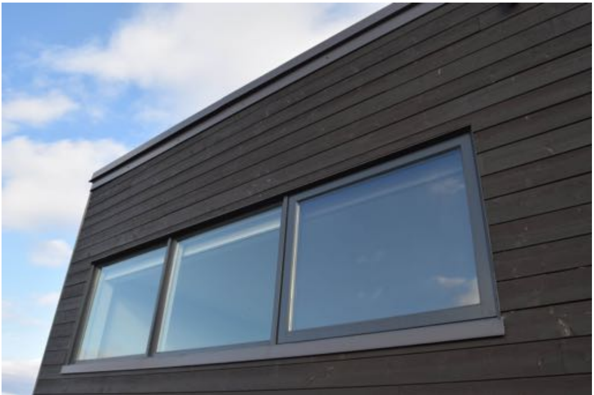
Photo 56: During the site visit walkthrough, a leak was reported at an elevated transom window, in the fourth floor den of unit 303.
