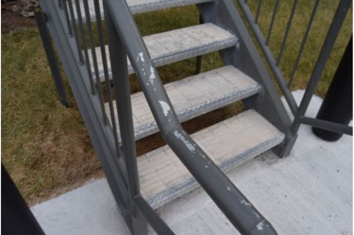
Photo 5: Paint is peeling on the south staircase railings and risers.
