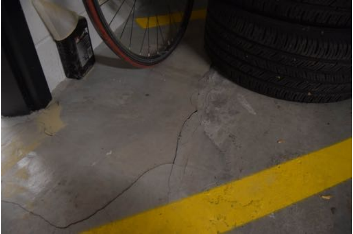
Photo 23: There are various size cracks in the cement slab at multiple locations.
