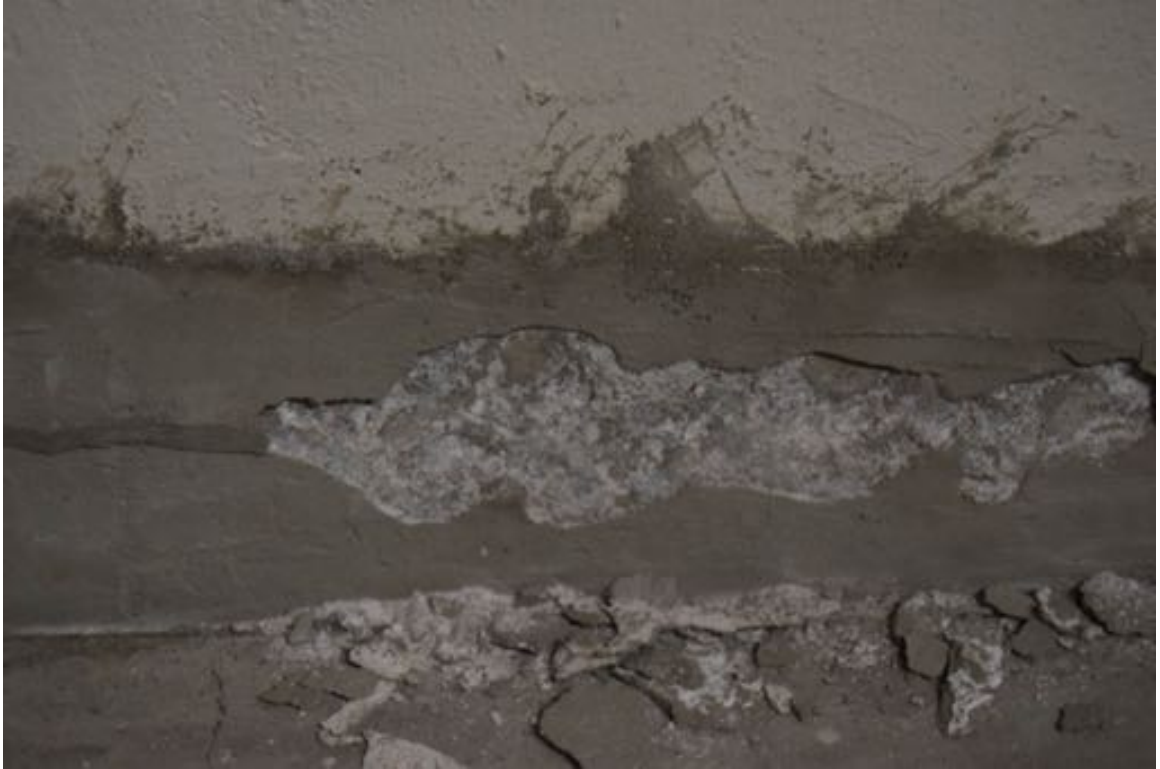
Photo 27: The parging coat on the foundation walls is deteriorating.
