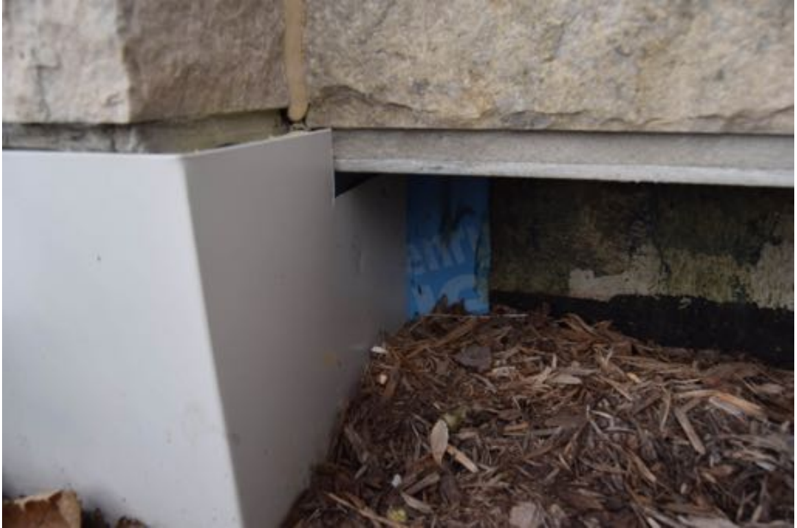
Photo 21: Northeast corner, portions of air/vapour membrane and primer visible near grade, under the stone veneer.
