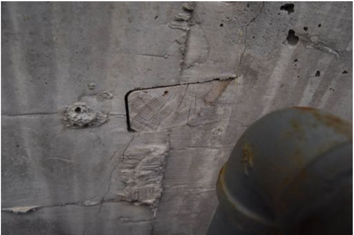
Photo 16: Southeast side, portions of form work remnants, and a wooden board visible at the foundation.
