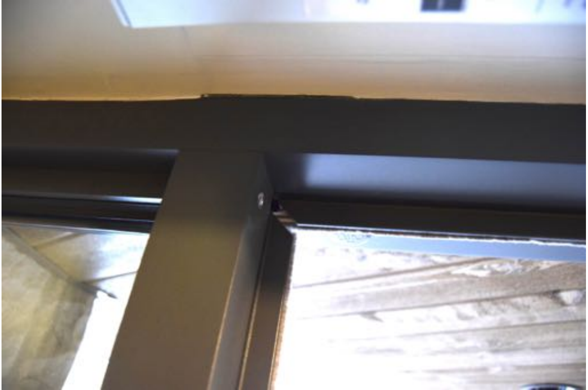
Photo 53: North lobby, there is a gap in the door frame visible.
