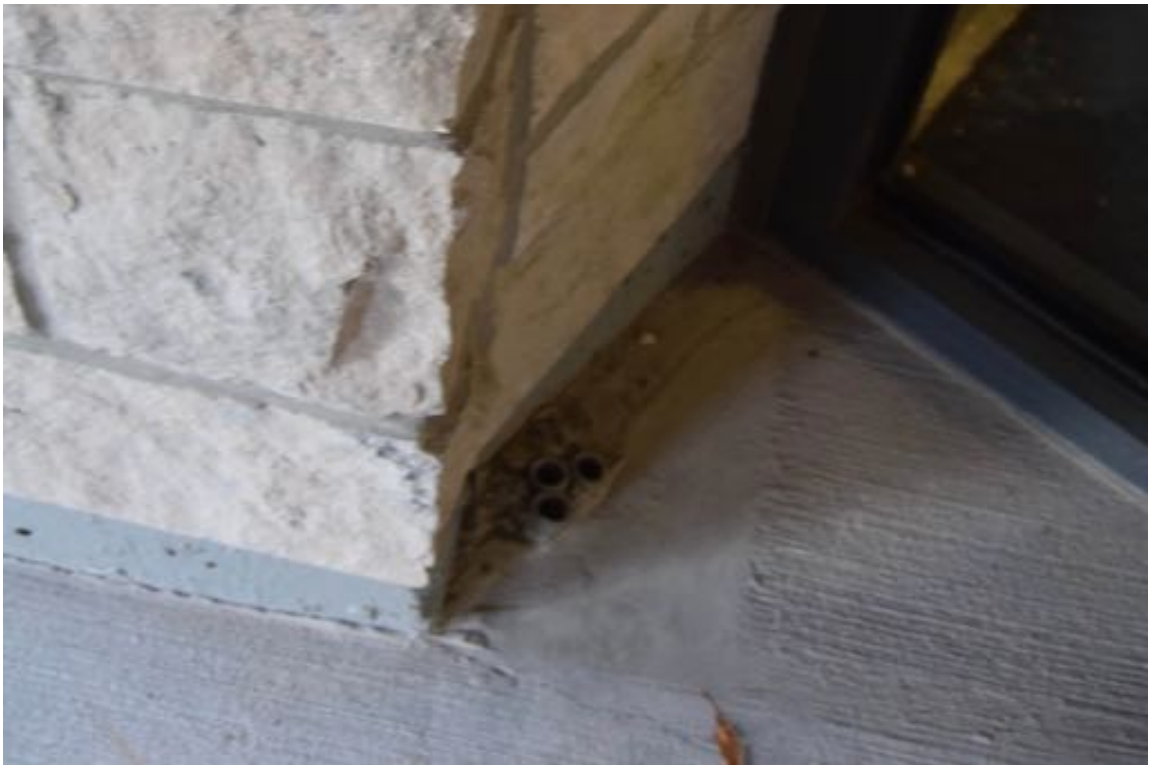
Photo 2: There are excess conduits visible in the concrete, near the left building entrance.
