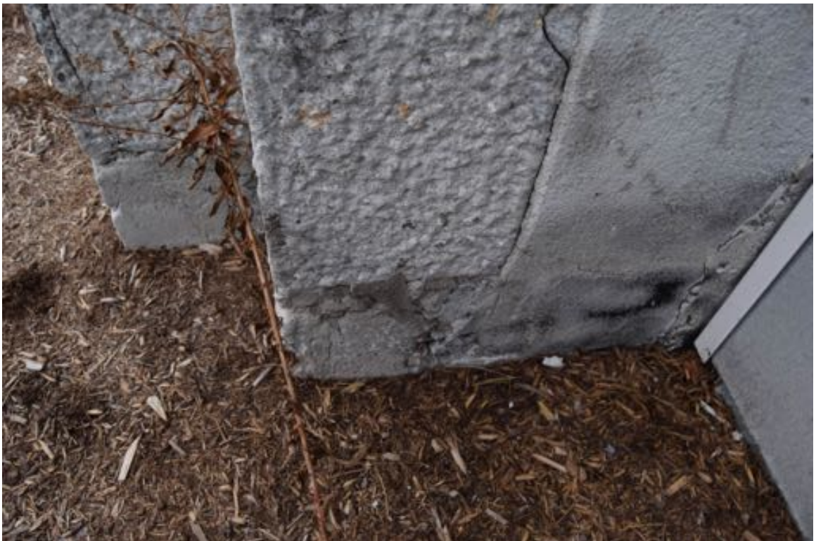
Photo 12: North elevation, near gridline E, portions of foundations under the existing stone veneer are deteriorating .
