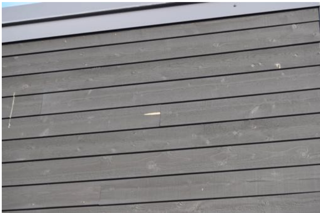
Photo 42: Wood siding is chipped on the wood cladding, at southeast common fourth floor terrace.
