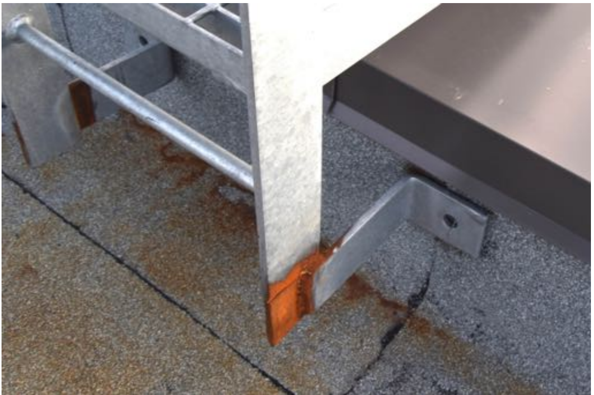
Photo 58: The metal access stairs to the main roof are not secured at the top .
