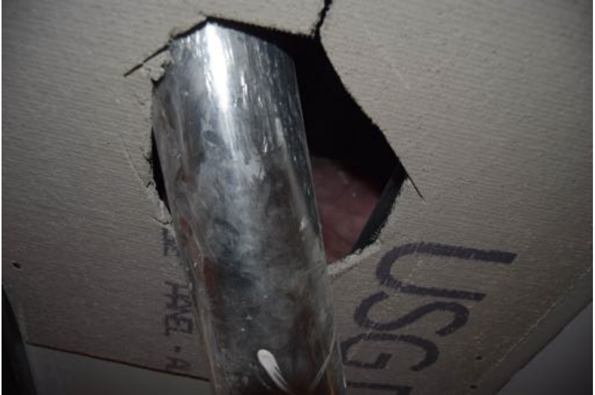
Photo 83: Ceiling panels near the unit heaters have gaps, with interior ceiling structure visible.
