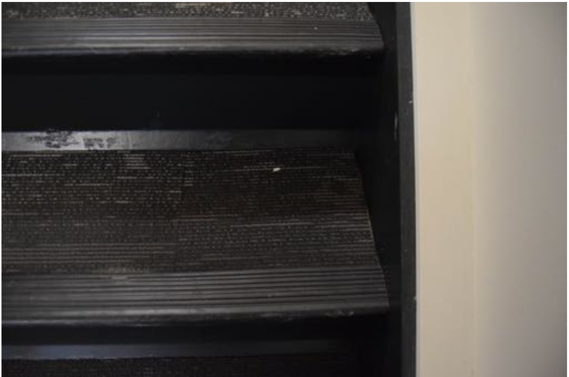
Photo 76: Multiple areas where the carpeted treads appear uneven.
