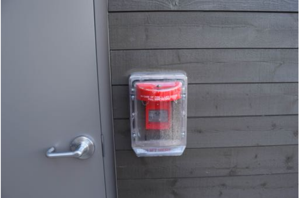
Photo 73: Condensation in the protective enclosure for a pull station at a fourth floor common terrace.
