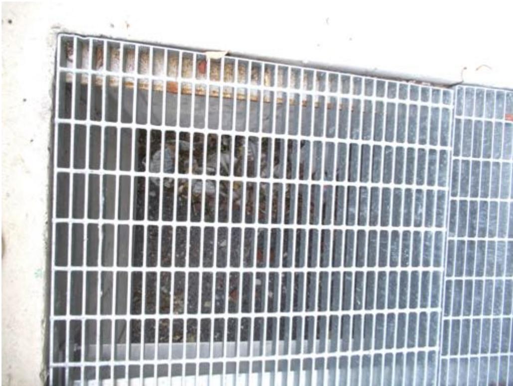
Photo 70: Construction debris/garbage should be cleaned out from the louvre shaft.
