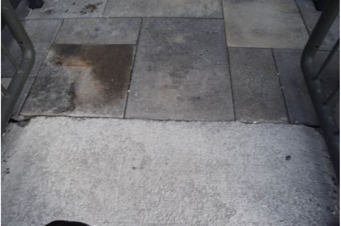
Photo 63: Multiple first floor terrace pavers are discolored at the walkway leading up to stairwell B entrance.
