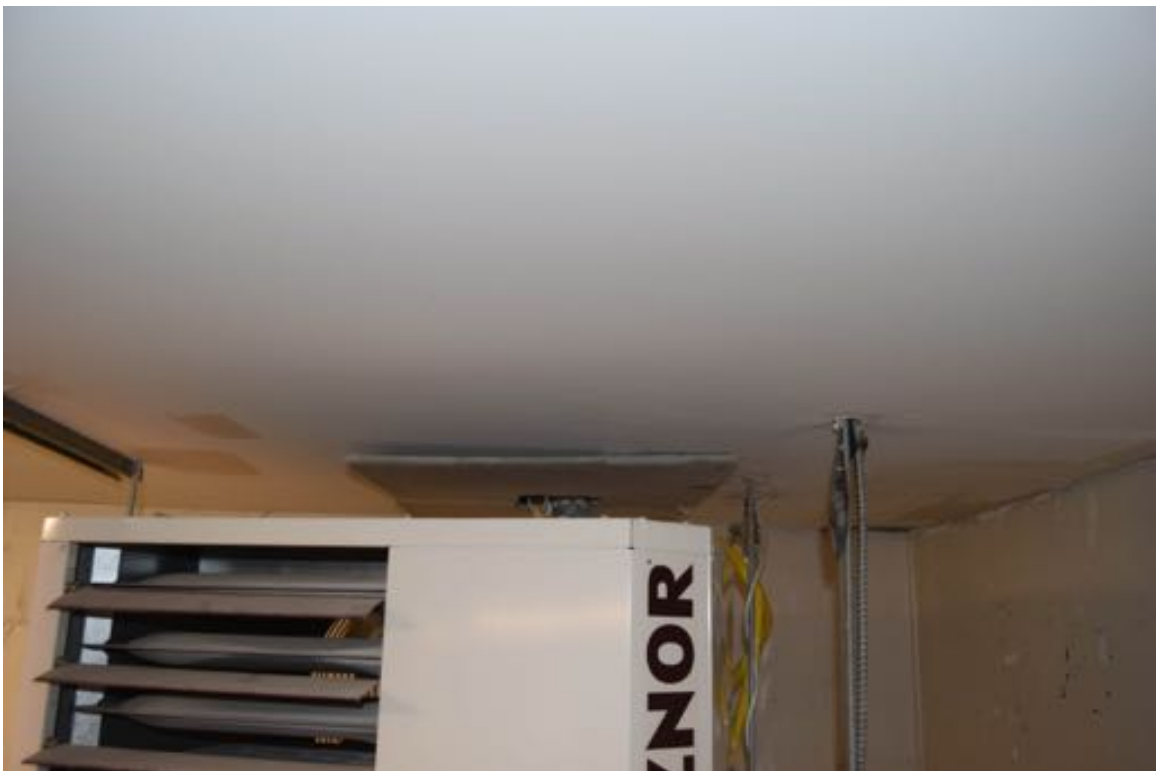
Photo 84: One of the ceiling panels near the unit heater is detaching.
