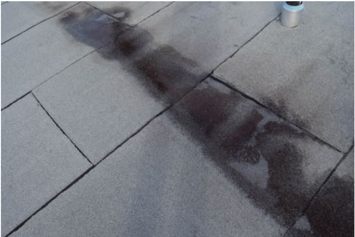
Photo 60: There is some evidence of standing water on the roof.
