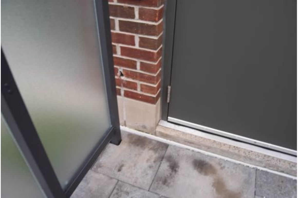
Photo 33: West elevation, hole in the brick veneer, near the entrance to stairwell B door.
