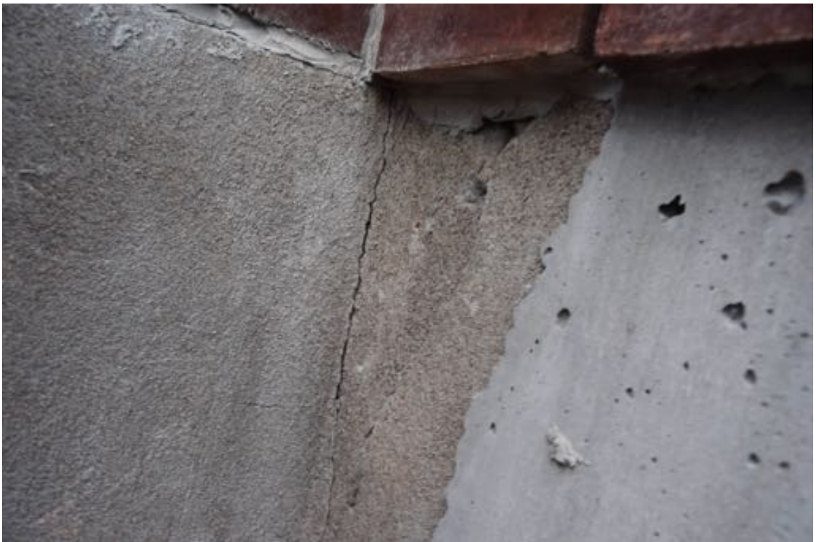
Photo 18: Southeast corner, multiple cracks noted at the existing foundation wall. This appears to be not new construction, not the 'exposed architectural finished concrete' specified in the architectural drawings.
