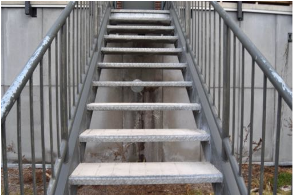
Photo 8: Paint is peeling on the north staircase railings, and risers.
