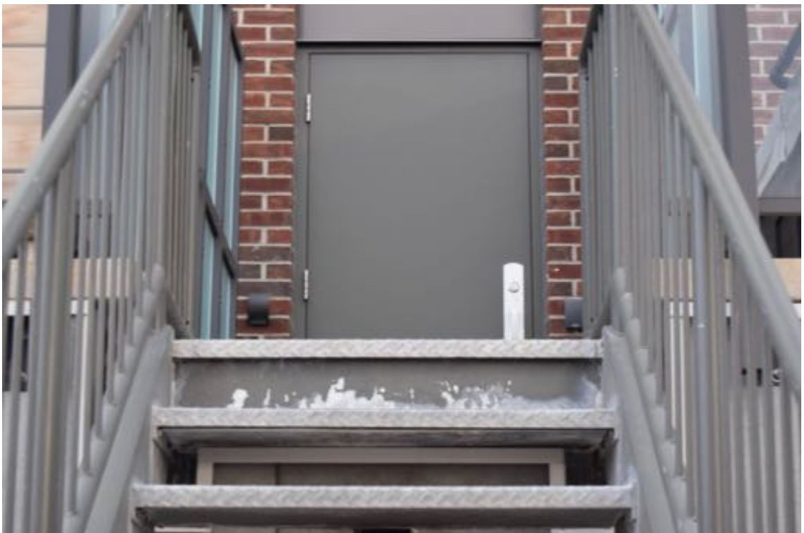
Photo 6: South staircase top riser is severely rusted
