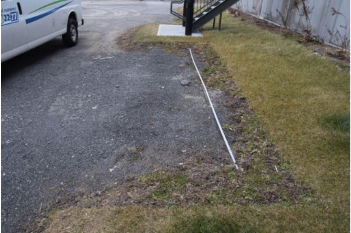
Photo 9: Sodded areas are incomplete at the rear west-end of the building, not as per provided drawings.
