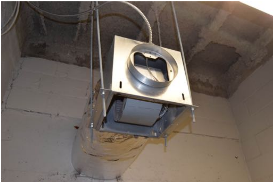
Photo 72: The garbage room ceiling-hung exhaust fan appears to have panels or ducting missing.
