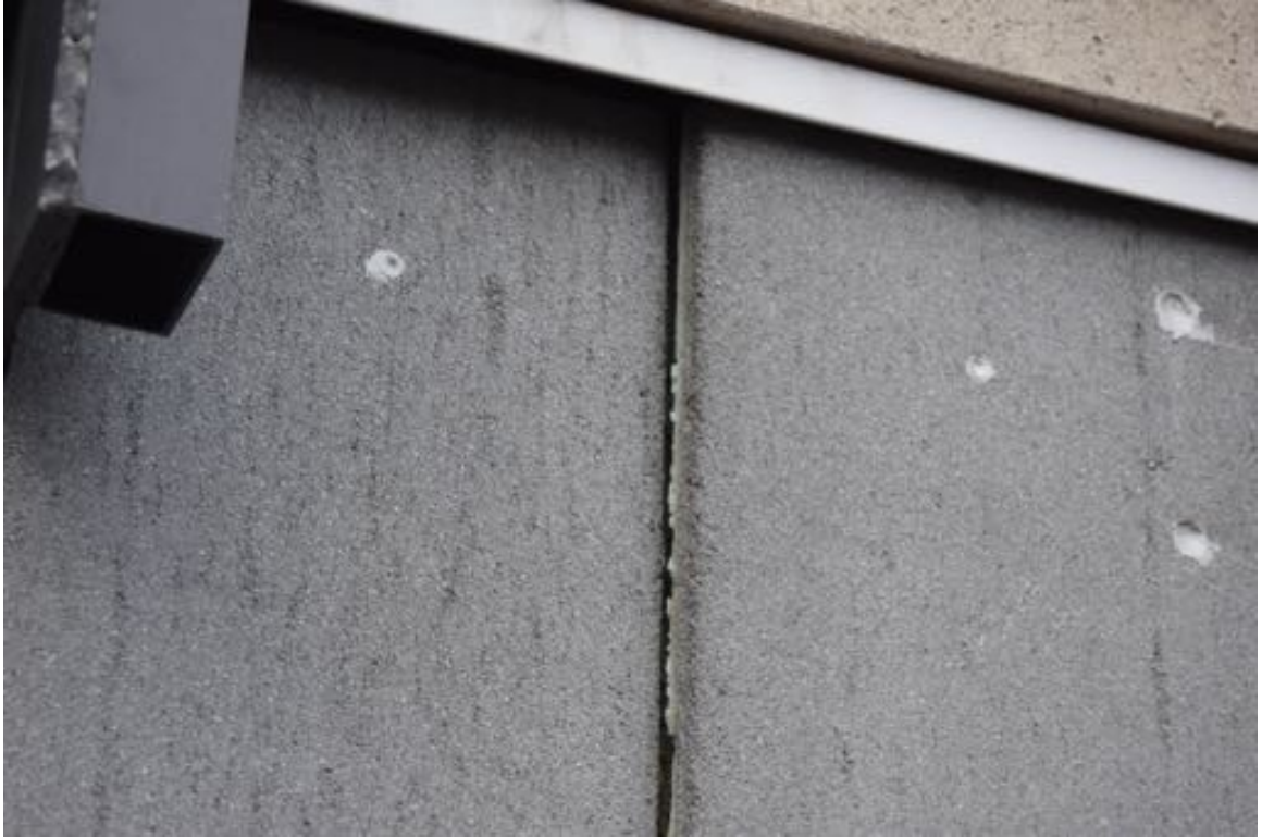
Photo 43: An insulation panel is dislodged at the southwest corner of the building.
