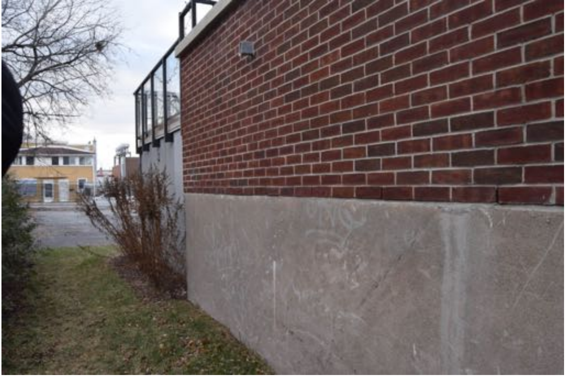
Photo 19: Multiple graffiti, scratch marks, and stains are also noted at this exposed foundation wall.
