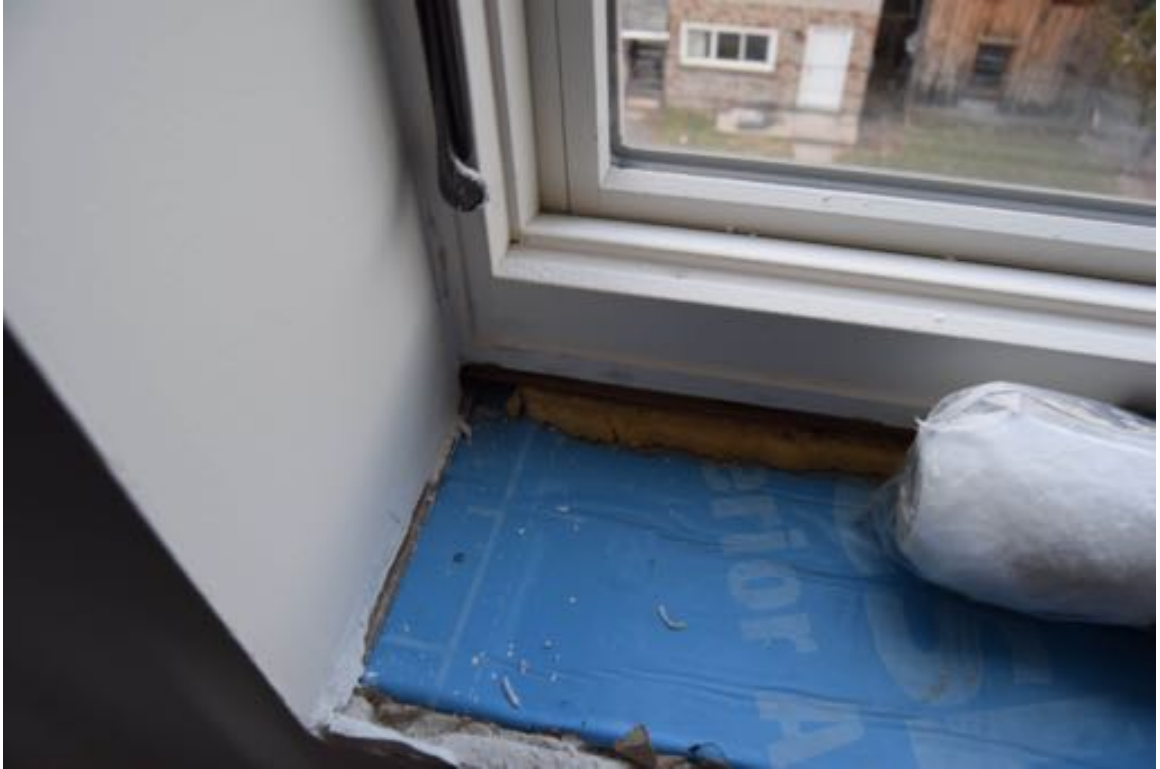
Photo 57: The windowsill was removed for repairs at a window reviewed at Unit 302, it is not clear if this was due to a leak.
