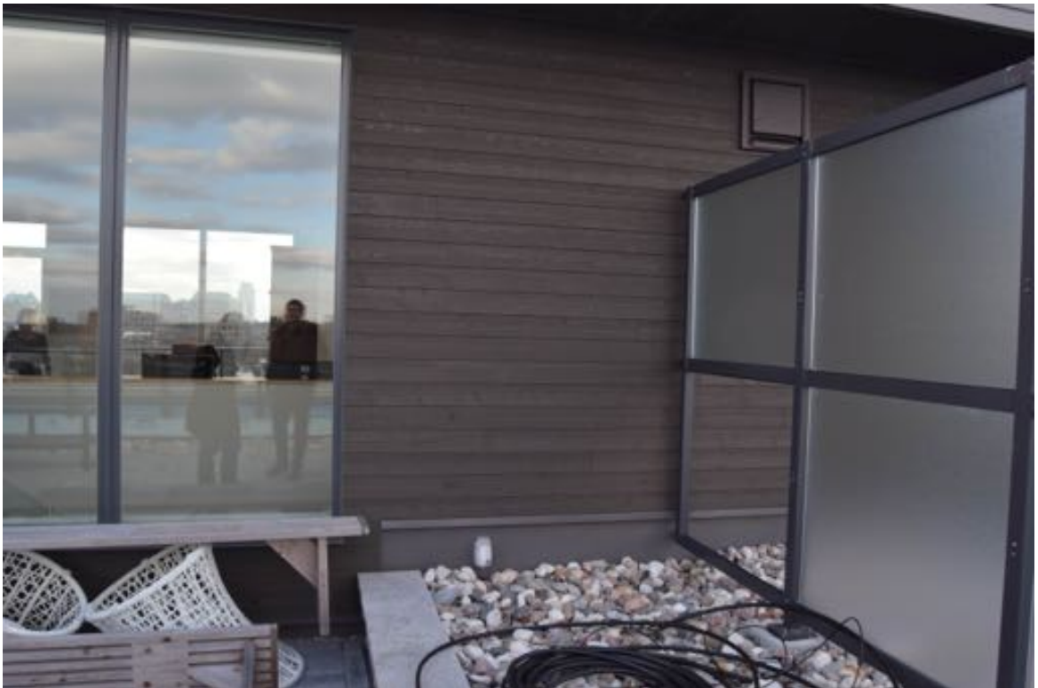
Photo 22: Glass panel piece missing in terrace privacy screen at Unit 302.
