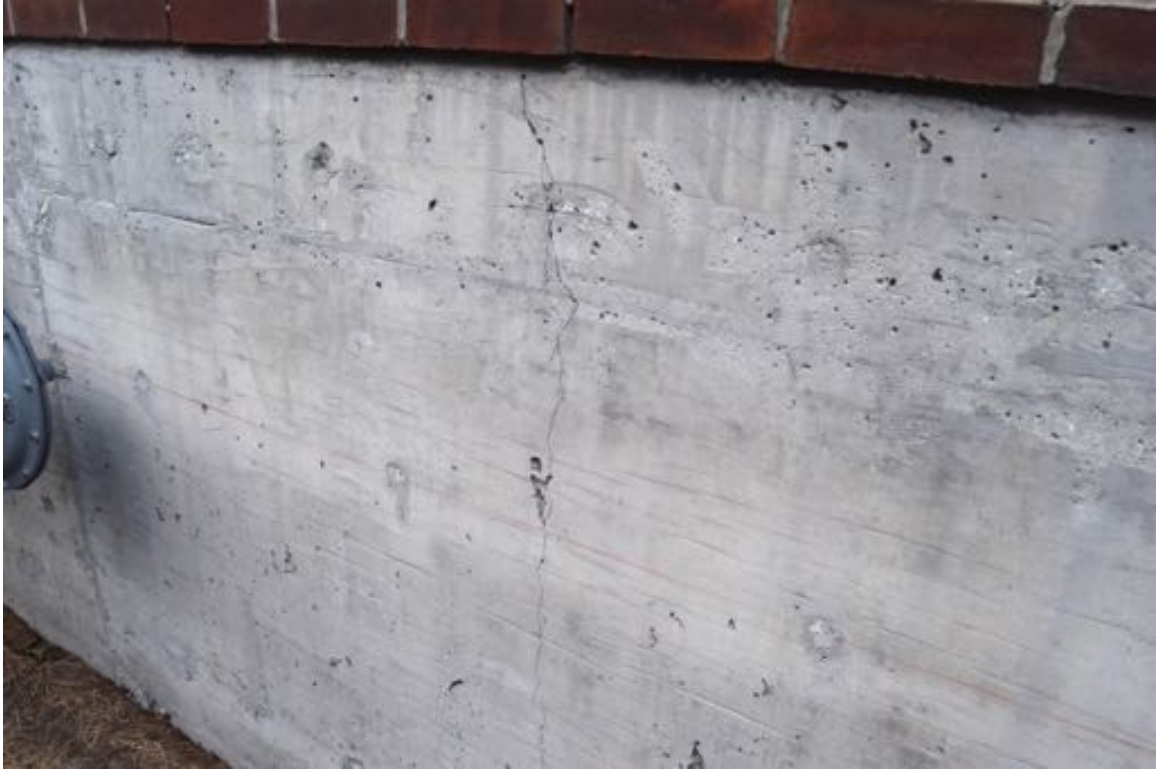
Photo 13: Southeast side of the building, a crack was noted on the exposed foundation wall.
