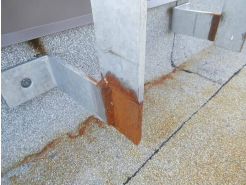
Photo 59: The metal access stairs appear to be rusting.
