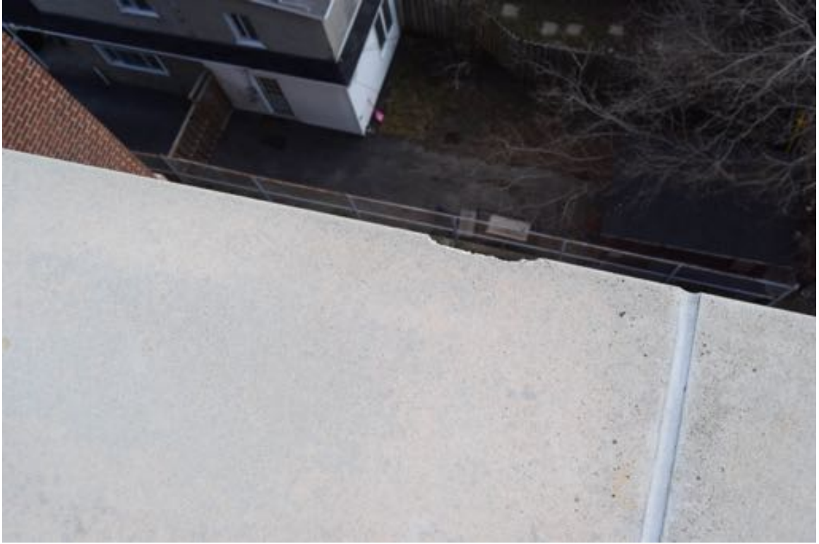
Photo 65: The fourth floor terrace parapet precast concrete caps are chipped.
