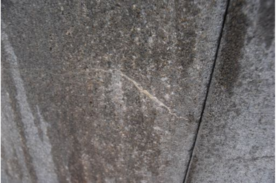
Photo 49: Multiple cracks are visible in the panels, particularly under the scuppers.
