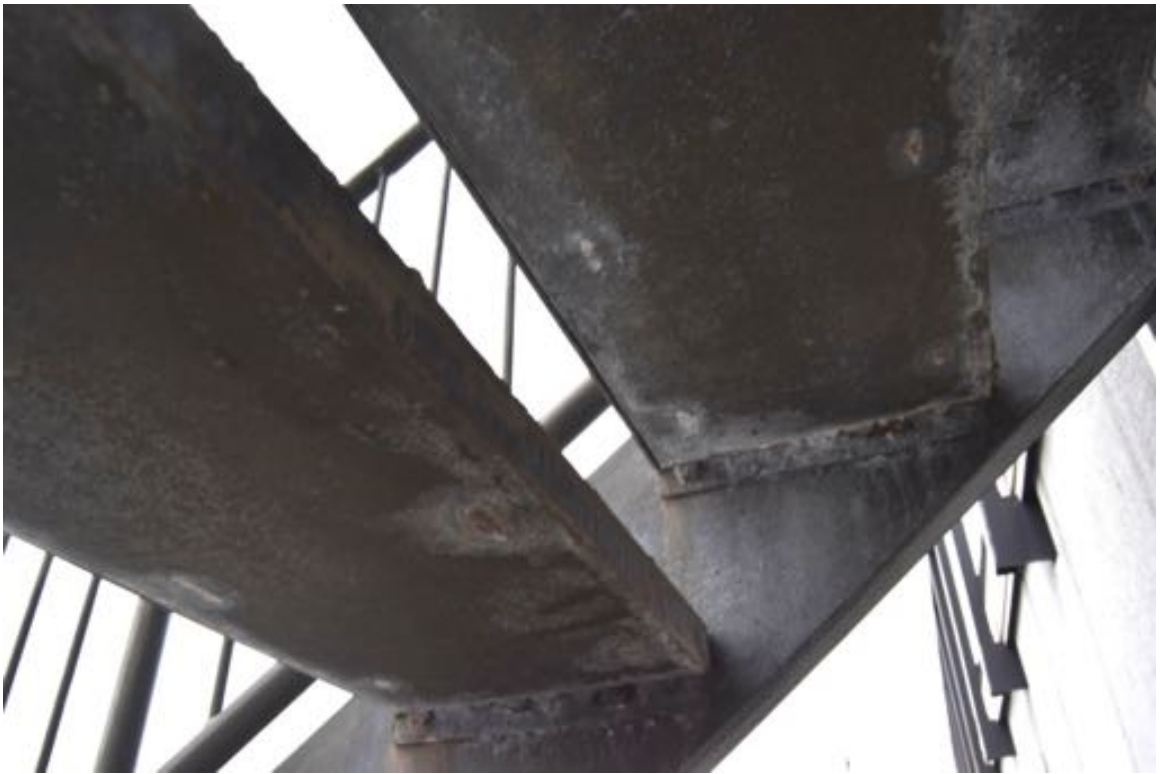
Photo 7: North staircase is rusting at the bottom.
