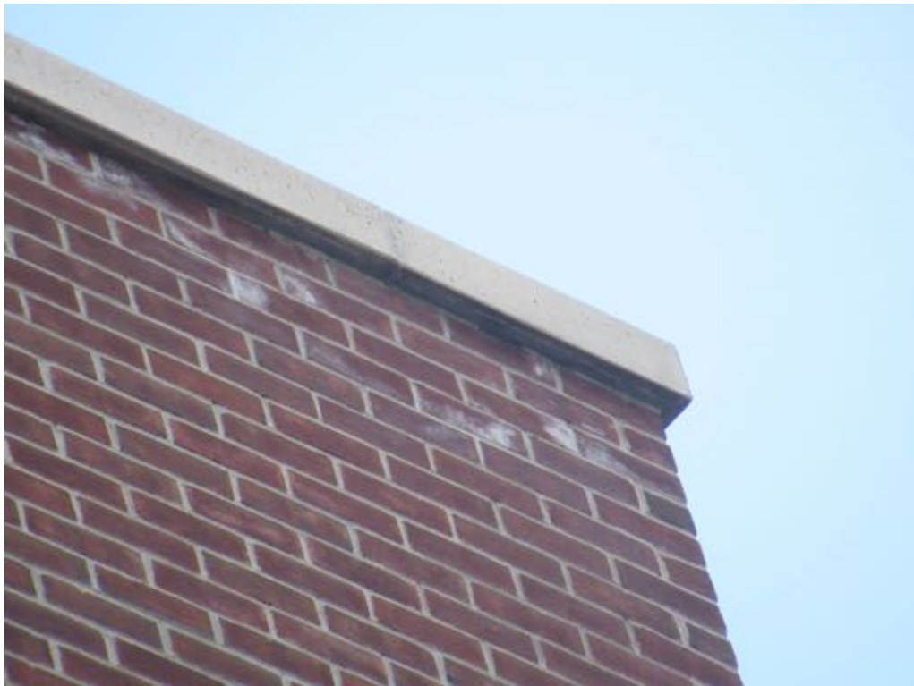
Photo 32: West elevation, discoloration/staining visible on brick veneer under rooftop terrace concrete precast tops.
