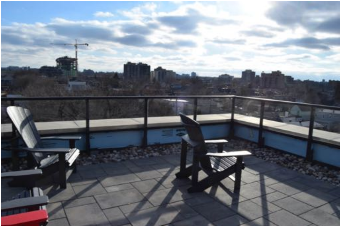
Photo 64: In multiple areas at the fourth floor terrace parapets, the metal flashing is missing, with the rigid insulation is exposed.
