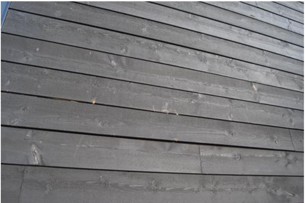
Photo 40: Various dings/scratch marks observed on the wood cladding, at northwest common fourth floor terrace.
