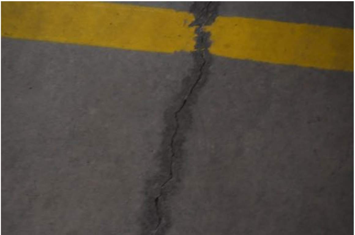
Photo 24: There are various size cracks in the cement slab at multiple locations.
