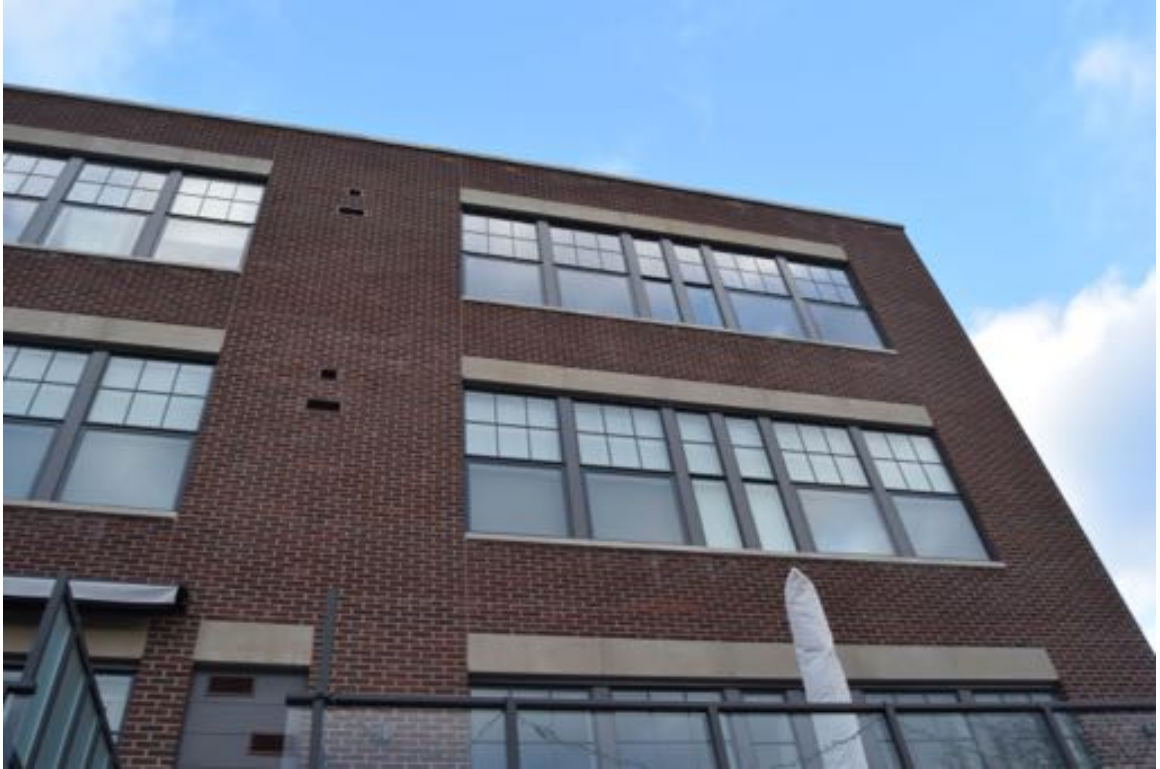
Photo 31: West elevation, discoloration/staining visible on brick veneer under numerous window concrete precast sills.
