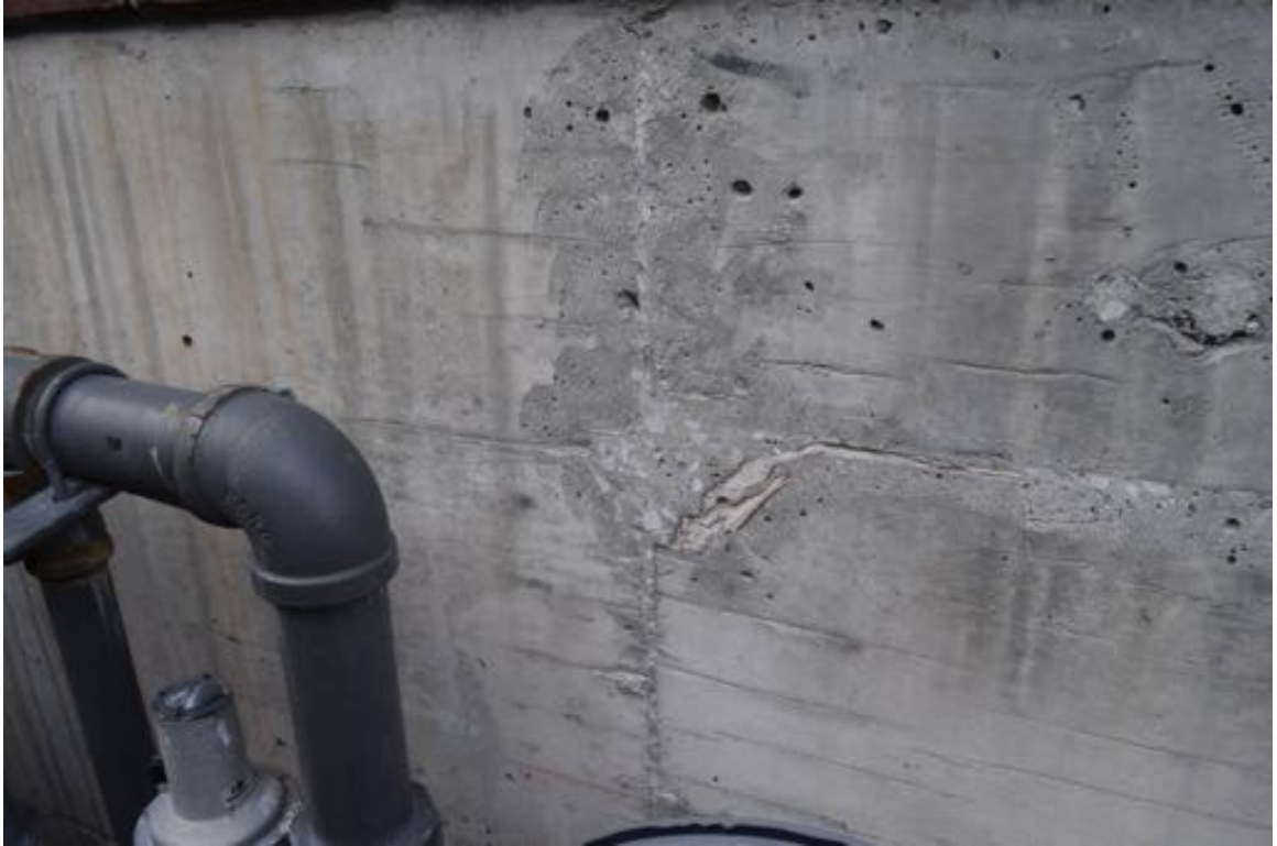
Photo 15: Southeast side, in general the foundation finishes are poor with remnants of formwork visible.
