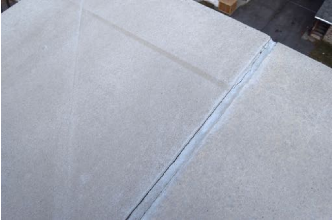
Photo 67: The mortar between the fourth floor terraces precast concrete caps is cracked, in multiple locations reviewed.
