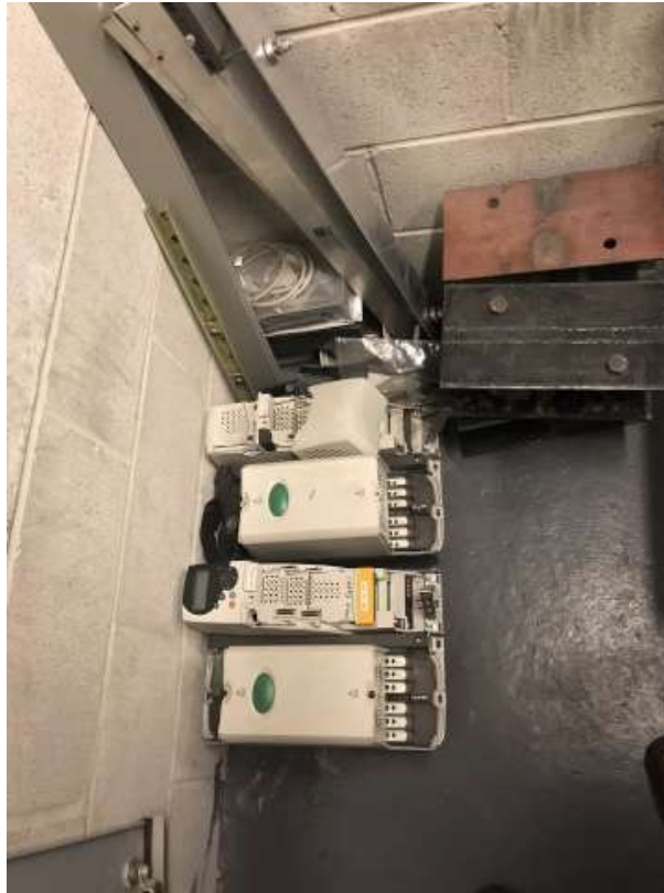
Photo 3: Spare parts in machine room - store properly
