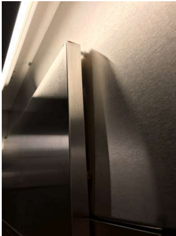
Photo 4: Applied car operating panel (#1) - properly align
