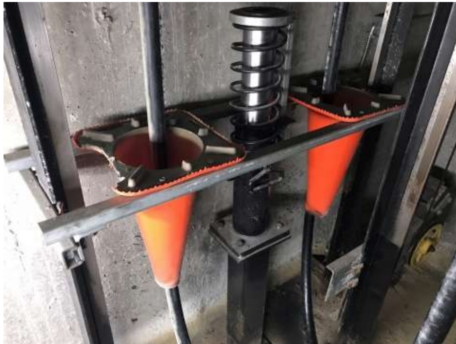
Photo 5: Compensation cable stabilizer (#1) - provide sufficient means
