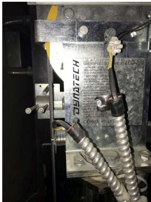
Photo 8: Governor (#2) - provide conduit
