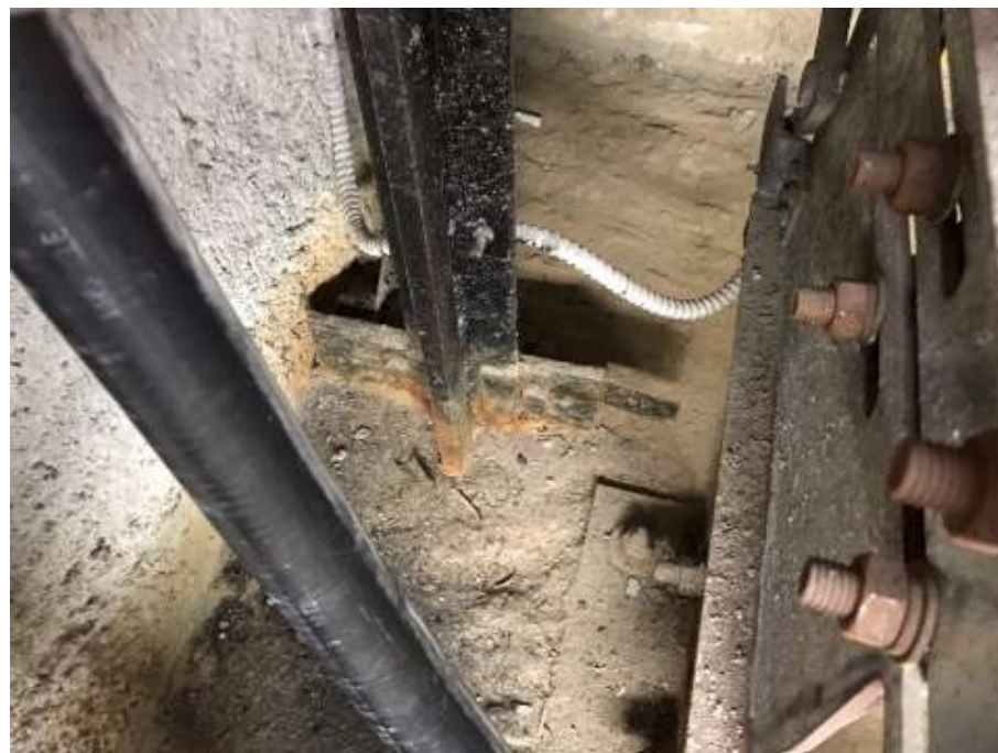
Photo 6: Counterweight pit steel (#1) - scrape and paint
