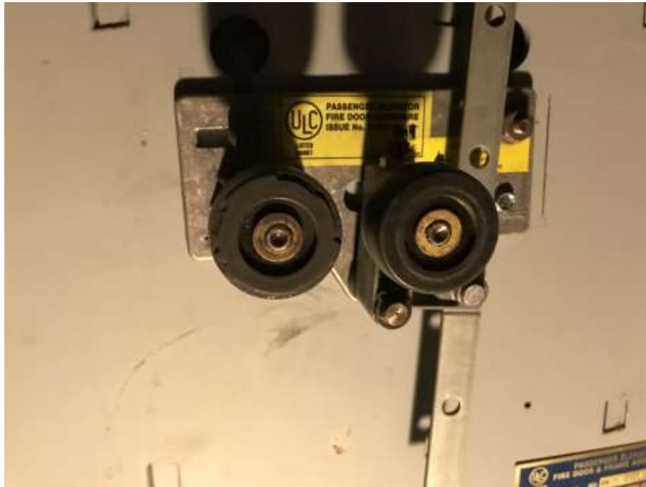
Photo 7: Hall pickup roller (#1) - replace
