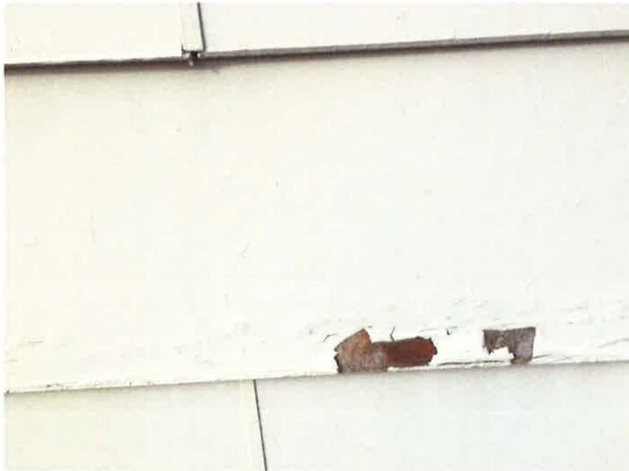
8 Showing existing hardboard siding to be replaced with vinyl siding
