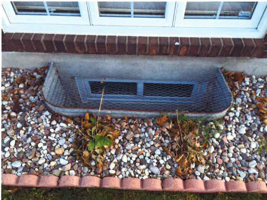
6 Showing a galvanized sheet metal window well
