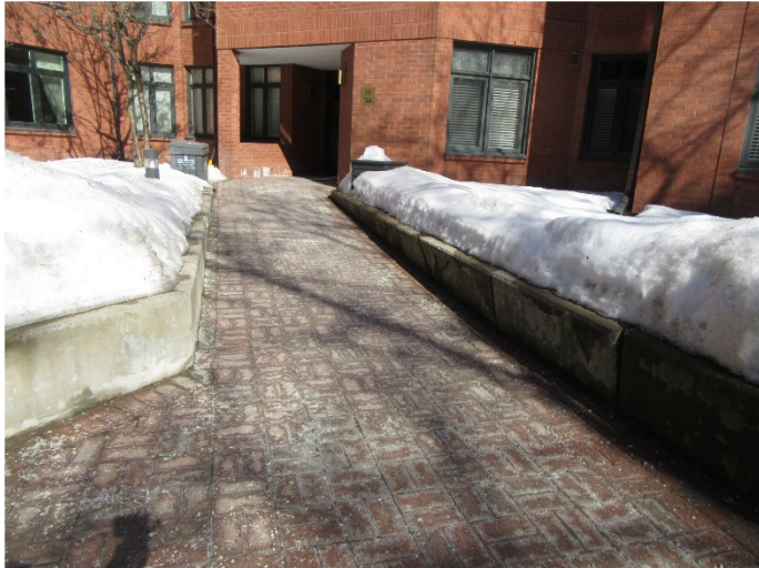
Photo D.3 – Showing precast concrete retaining walls that are leaning.
