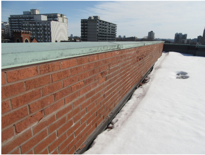
Photo D.5 – Showing numerous spalled brick at a parapet wall.
