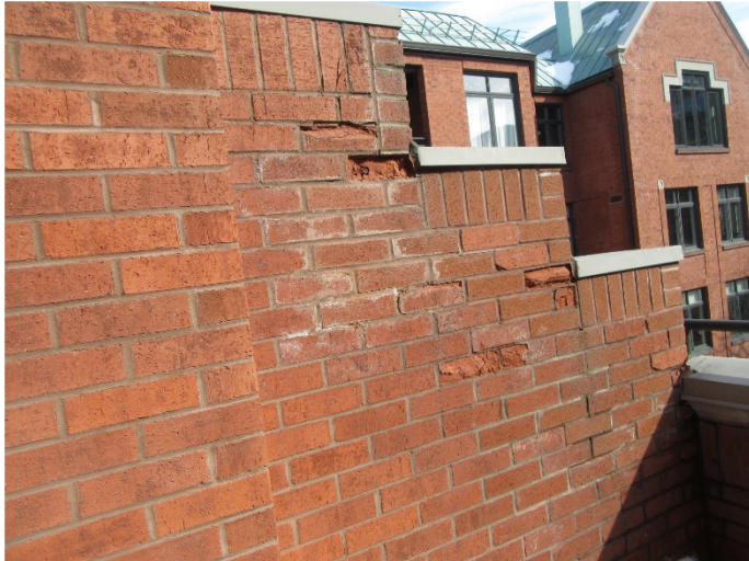
Photo D.7 – Showing a spalled bricks at a balcony privacy wall.
