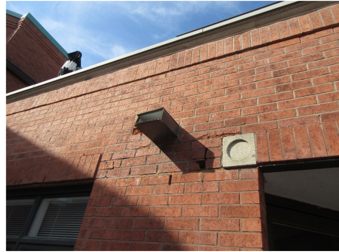
Photo D.6 – Showing spalled bricks near a balcony scupper.
