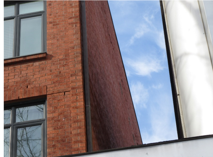
Photo D.8 – Showing numerous spalled bricks at the east elevation.
