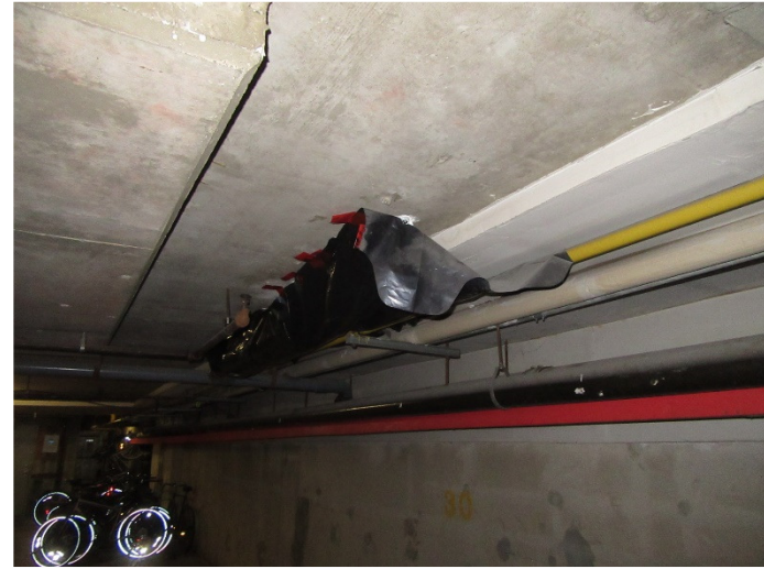
Photo D.2 – Example of a leak through the podium deck membrane into the parking garage.
