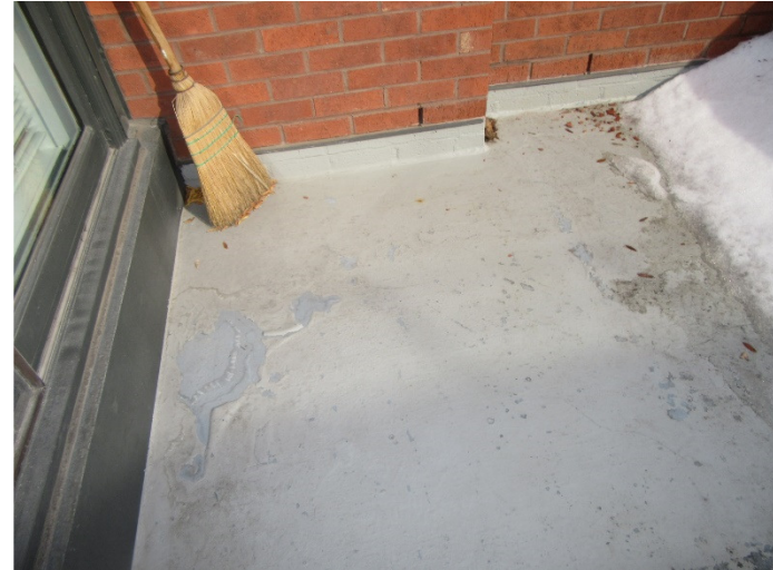
Photo D.4 – Showing balcony waterproofing membrane that is peeling.
