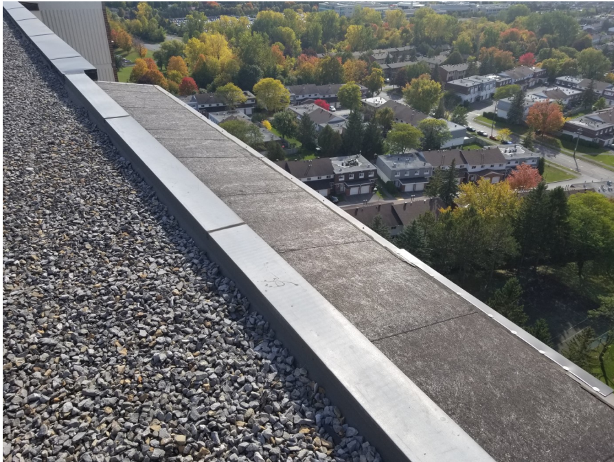
6 Recently replaced conventional balcony canopy roof
